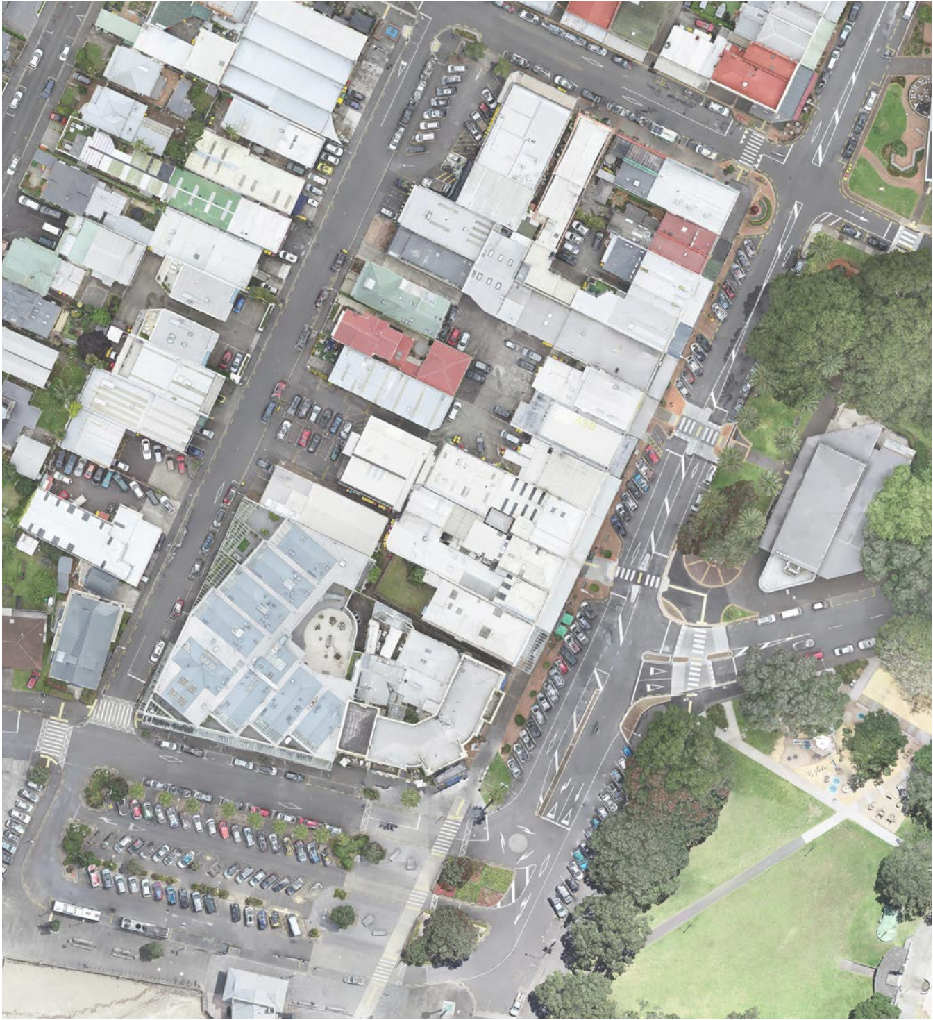
Survey Aerial View of Block, Devonport
