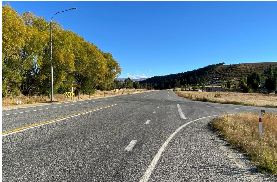
Photograph 4: State Highway 6 / Lowburn Valley Road Intersection (Looking South)
