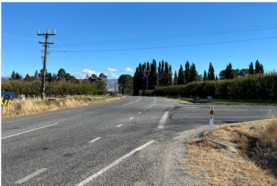
Photograph 5: State Highway 6 / Burn Cottage Road Intersection (Looking South)
