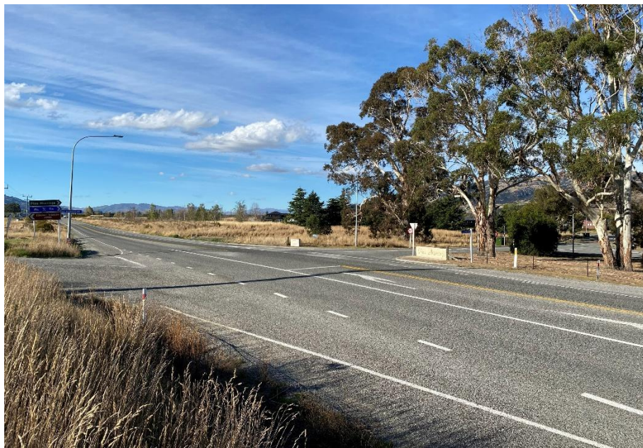
Photograph 3: State Highway 6 / Pisa Moorings Road / Clarke Road Intersection (Looking North)
