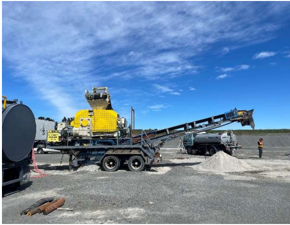
Photograph 1: View of the HRC™800 crushing plant and showing a small stockpile of crushed gravel.
