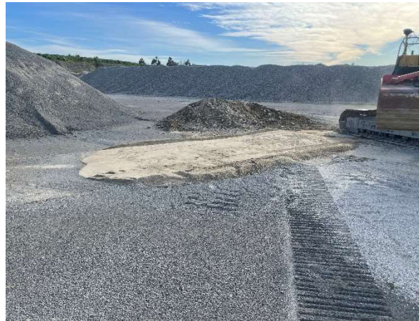
Photograph 4: View of the prepared base prior to formation of the trial hardfill pads.
