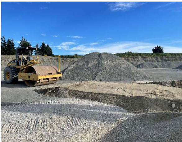
Photograph 5: Trial pad 1 prior to compaction.
