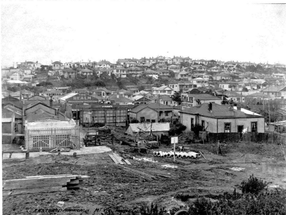
Figure 37 - Preparation of site at Hataitai (Clear area in foreground is now corner of Ruahine & Taurima Streets) 84
