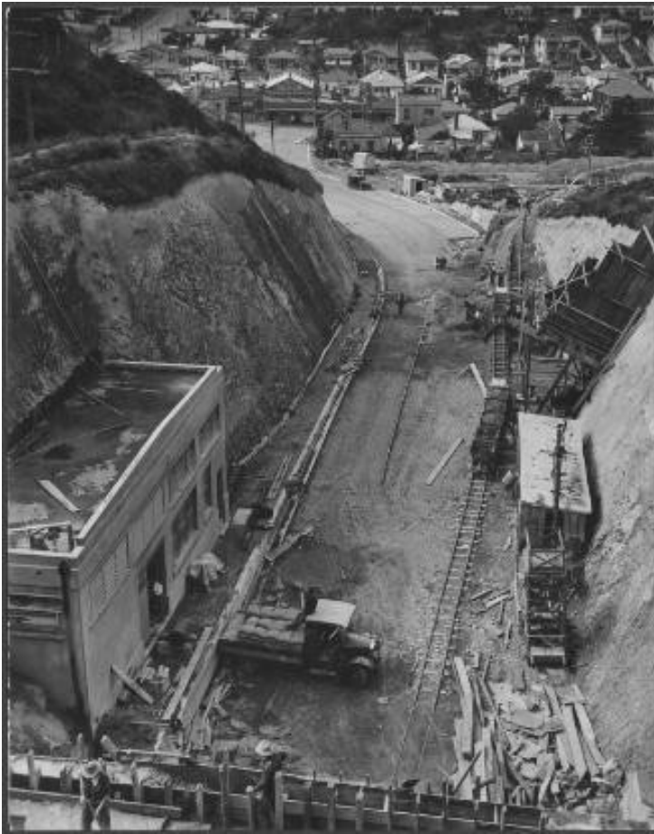
Figure 44 - View of the approach from Hataitai to the Mount Victoria Tunnel: March 1930 92
