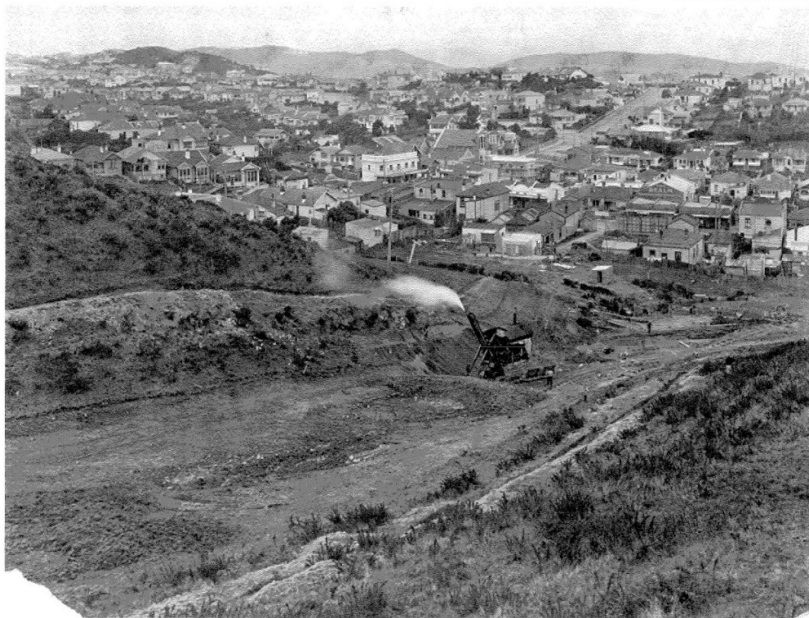
Figure 42 - Initial excavations on Hataitai side 89
