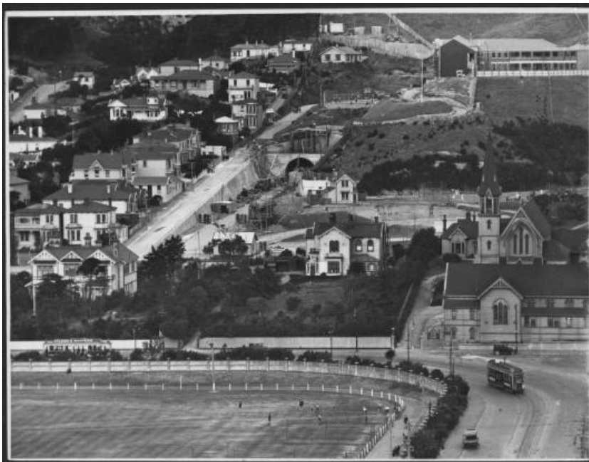
Figure 40 - View of the western entrance of the Mount Victoria Tunnel under construction, August 1930 87
