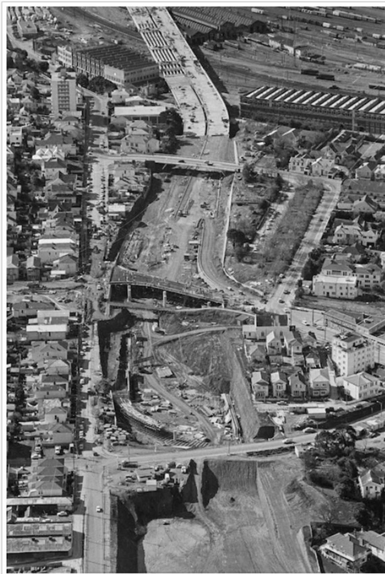
Figure 7 - Wellington motorway under construction 24
