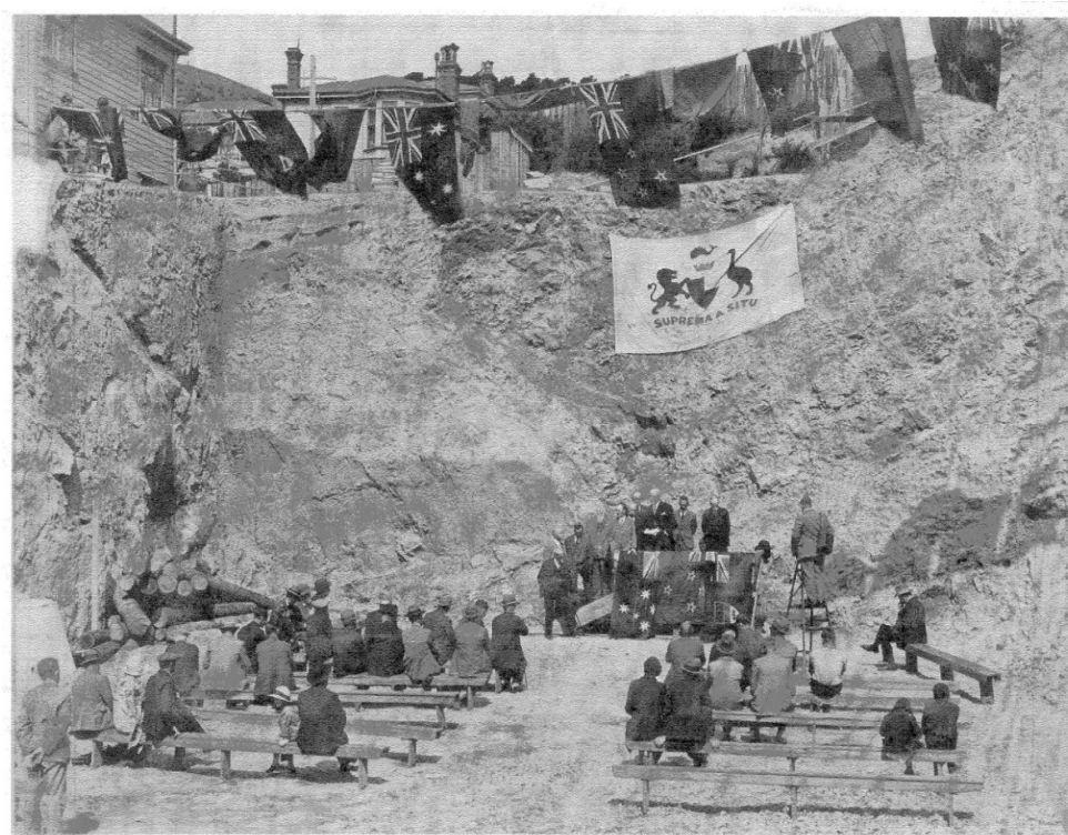
Figure 38 - Rock breaking ceremony, Mt Victoria side, December 1929 85
