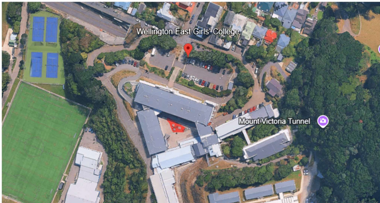
Figure 37 – Buildings in the Mt Victoria Tunnel West Area
