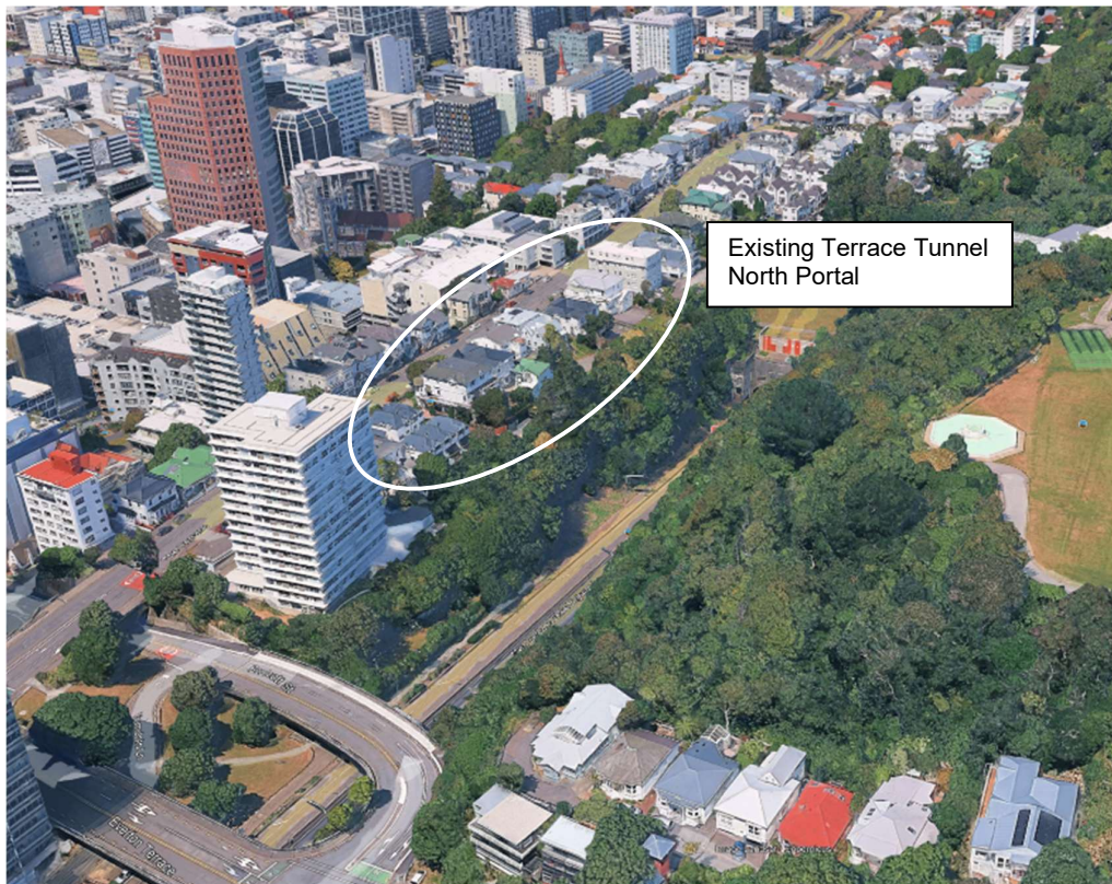
Figure 26 – Properties above the northern approach to the Terrace Tunnels
