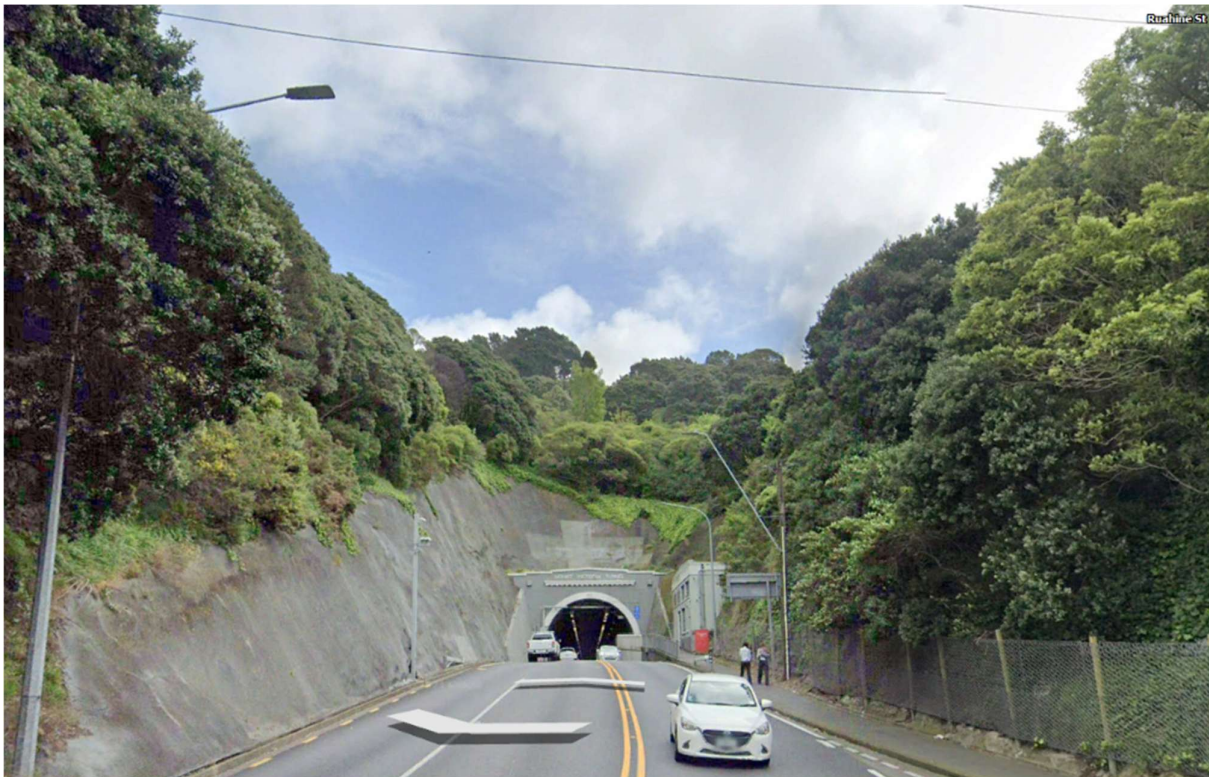
Figure 24 – Shotcrete surfaced slopes above eastern approach to the Mt Victoria Tunnel
