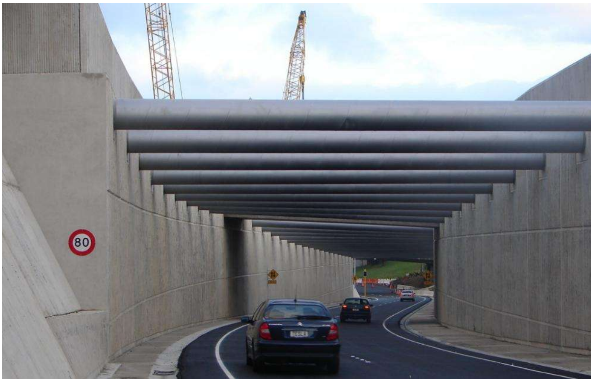
Figure 51 – Similar existing propped trench at the Inner City Bypass, south of the Terrace Tunnel
