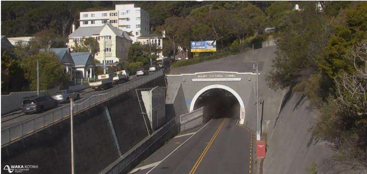
Figure 53 – Oblique view of the Western Approach to the Mt Victoria Tunnel
