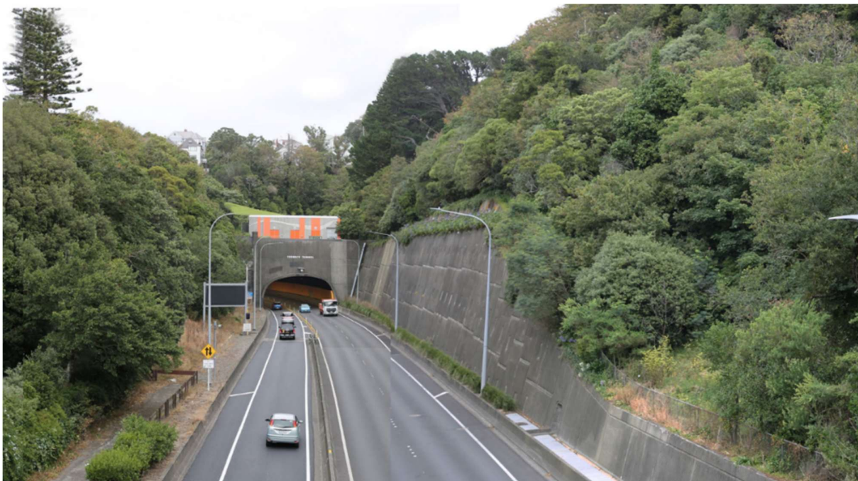
Figure 23 – Retaining wall and slopes above northwestern approach to the Terrace Tunnel
