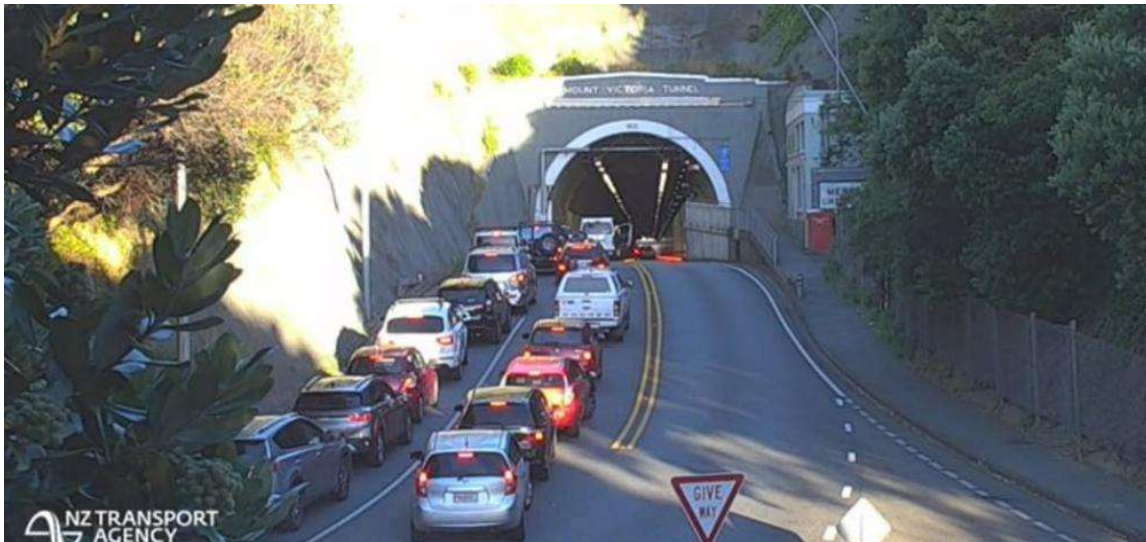
Figure 59 – Oblique view of the Eastern Approach to the Mt Victoria Tunnel
