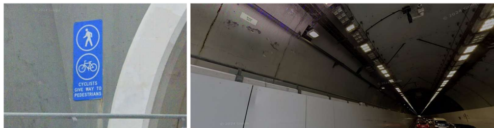
Figure 10 – Shared path through Mt Victoria Tunnel and signage
