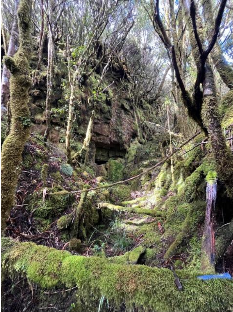
Figure 12. Looking along the tramway cutting to the main drive of the Koranui Mine
