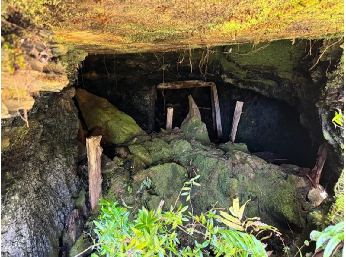
Figure 39. Mine portal with standing timber bracing (Feature 108)
