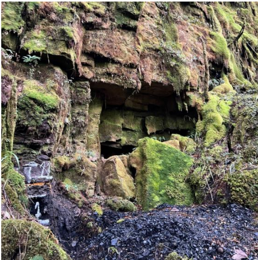
Figure 11. The collapsed entrance to the main drive of the Koranui mine at the top of the horse tramway. Coal debris is piled in front of the entrance
