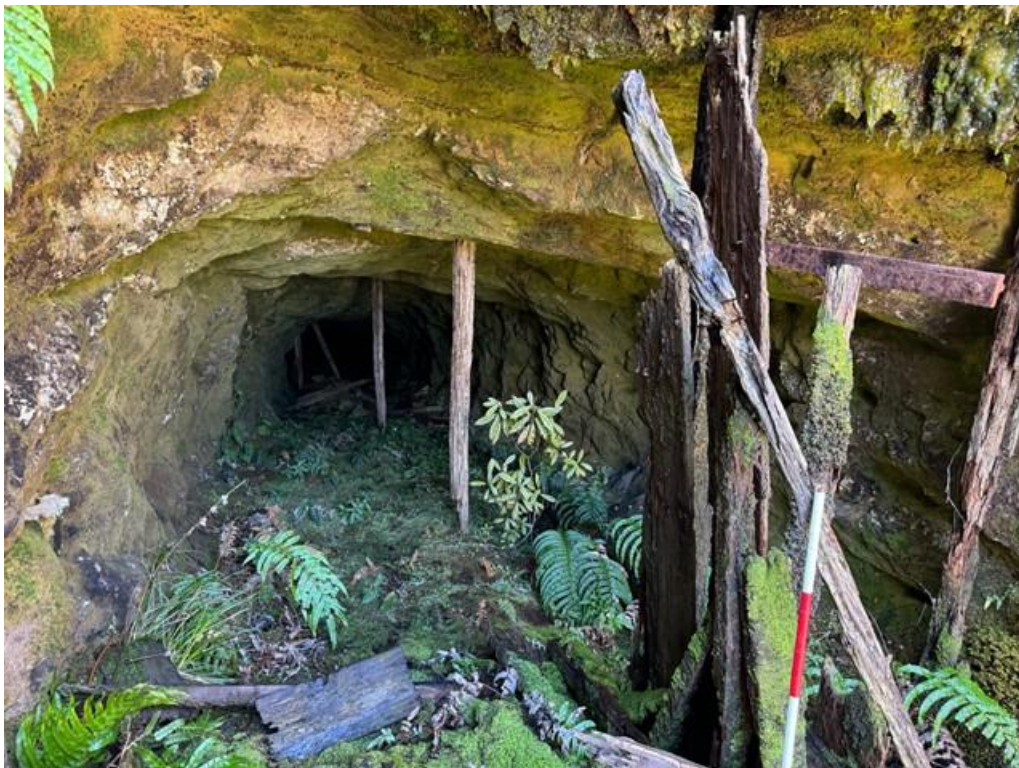
Figure 28. Entrance to the Taipo Mine stone drive with standing and collapsed timber bracing (Feature 131)
