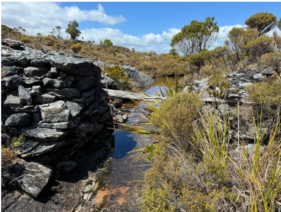
Figure 26. Stacked stone buttresses and the remains of the tramway bridge from the upper Taipo Mine area to Kiel's Flat (Features 133 and 132)
