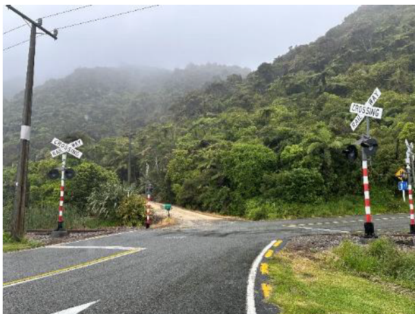
Figure 3-3: Western approach to level crossing from SH67
