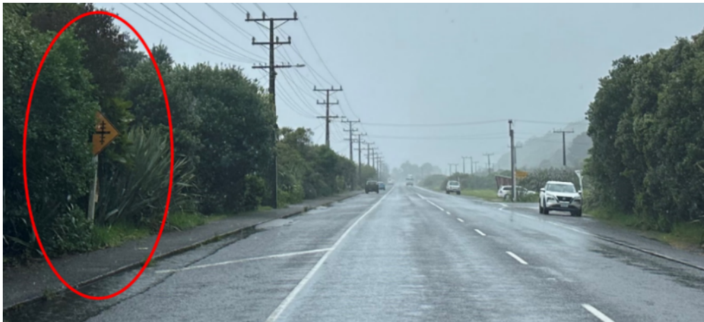
Figure 3-17: WXR2 sign on approach from south of SH67 hidden behind vegetation
