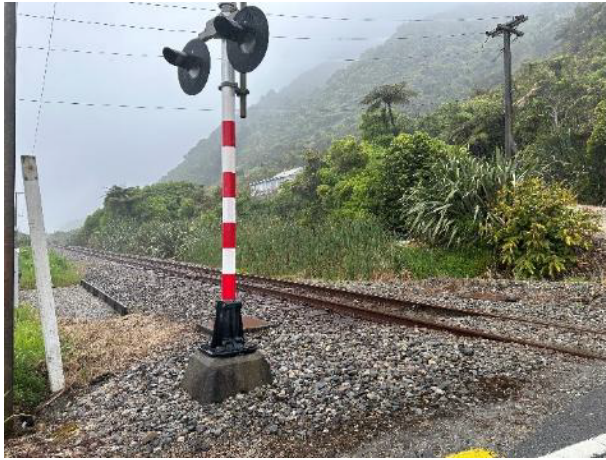
Figure 3-5: UP track sightline on western approach
