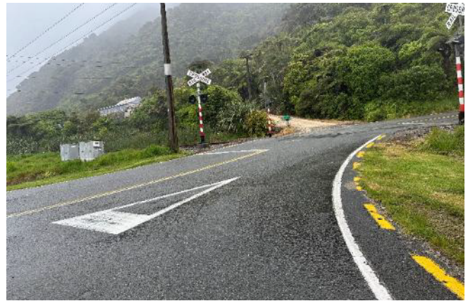
Figure 3-16: Steep gradient on western approach
