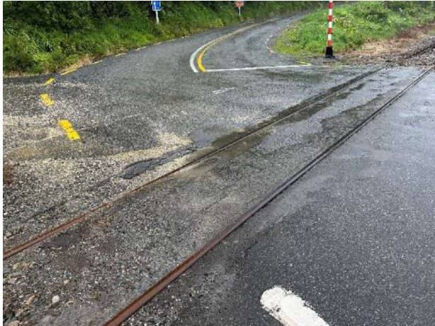
Figure 3-9: Track panel is breaking up
