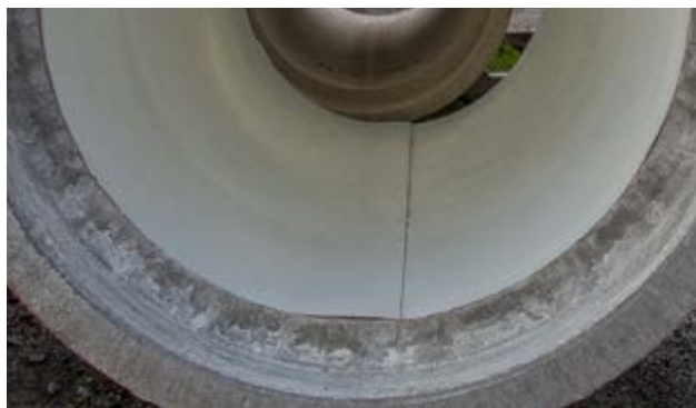
FIG. 1 Where 360° cover is required, the liner is fitted with an overlap at the invert (50 mm min)
