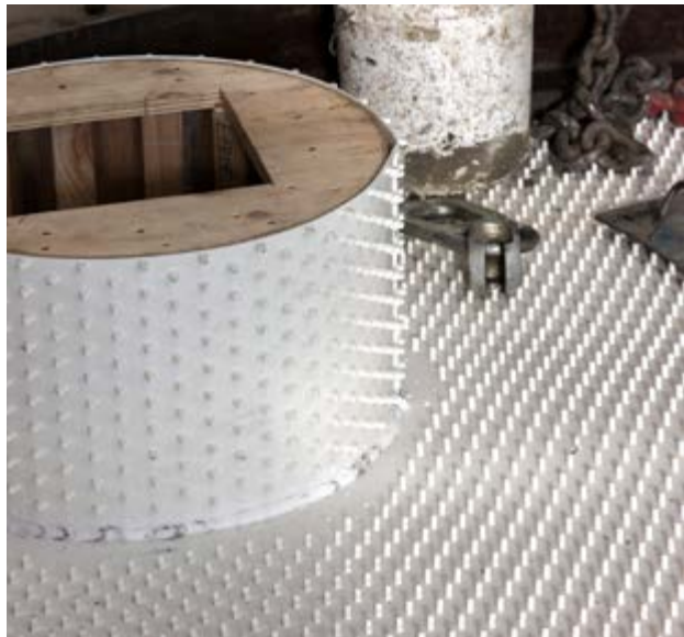
FIG. 14 Liner being installed for a manhole lid
