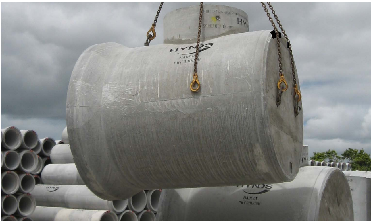
FIG. 6 Point lift of typical plugged end pipe
