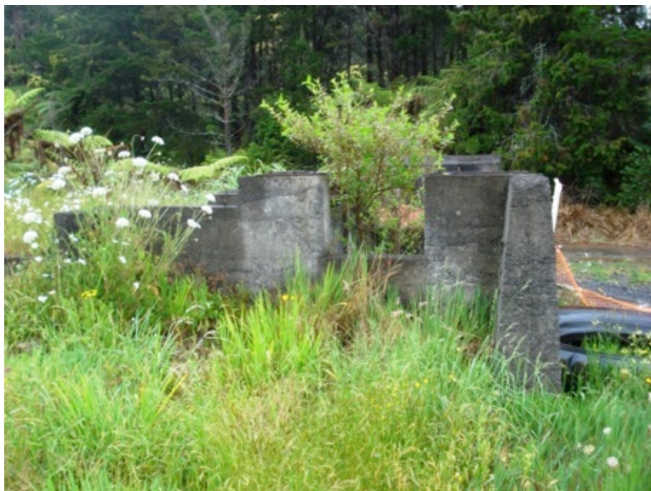
Mineral Resources crusher foundations.
