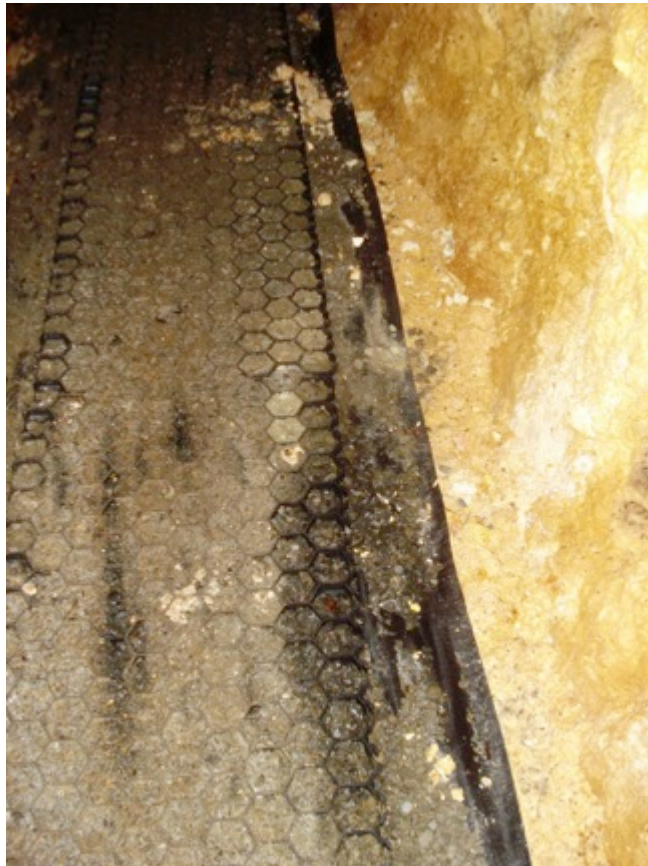
Plastic Paving in the Collins Drive, Tairua.
