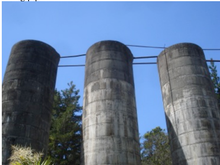
Ferro-concrete tanks.
