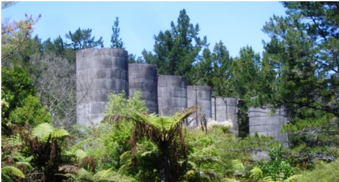
Ferro-concrete Cyanide tanks. Union Hill 2012. Photo: E.T.Coppard.
