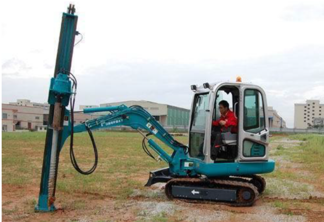
Figure 8. Example of screw pile driving method to be used on site. (Source: FNSF, 2025).
