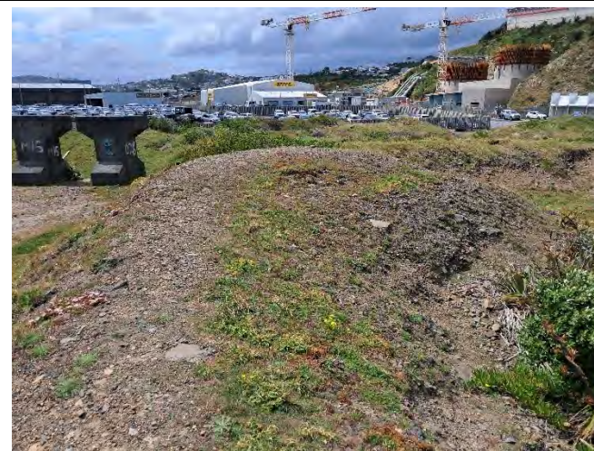
Photo 6. East side of the seawall, facing north-east towards the Moa Point WWTP.
