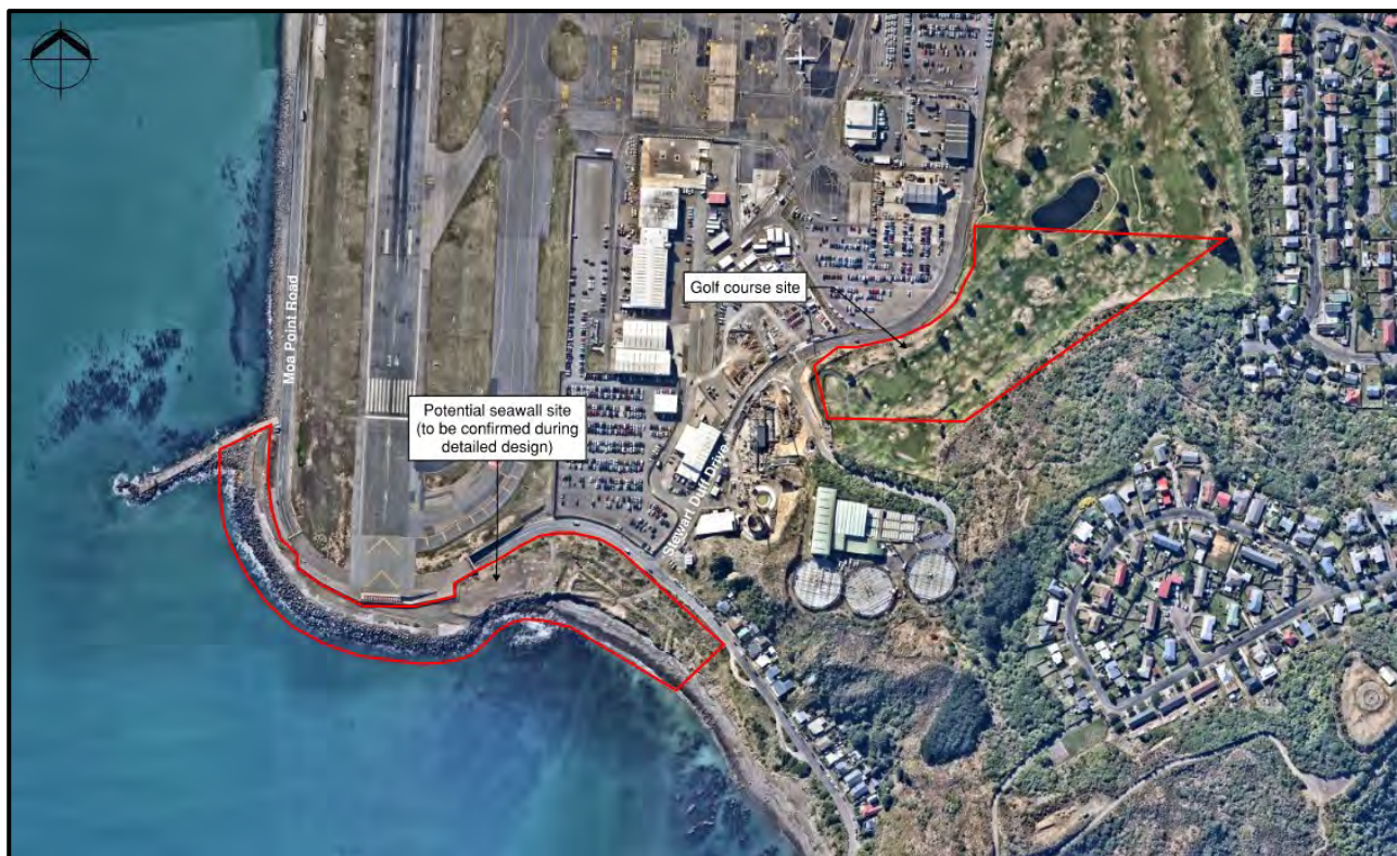
Figure 2. Site extent in the red polygons as of November 2024 (Source: NearMap)
