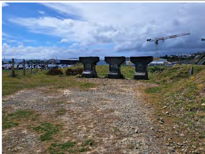
Photo 5. East side of the seawall, facing north.
