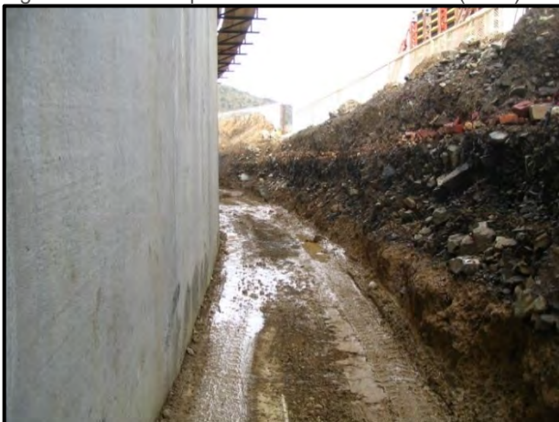
Figure 12. The soil profile on the south side of the tunnel
