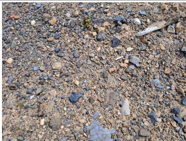
Photo 2. Composition of fill at surface on the seawall
