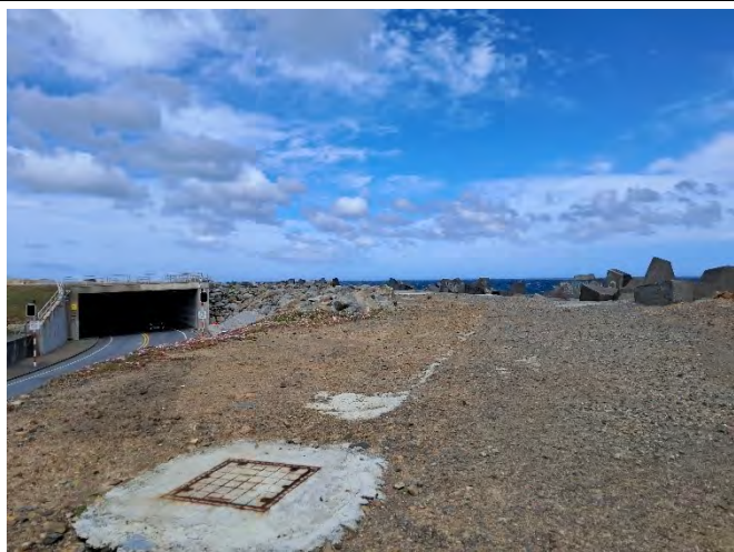
Photo 1. View from the west end of the seawall. Moa Point Road tunnel is visible far left.
