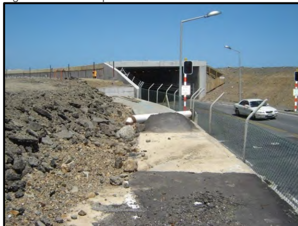
Figure 13. The constructed tunnel (24 November 2006)
