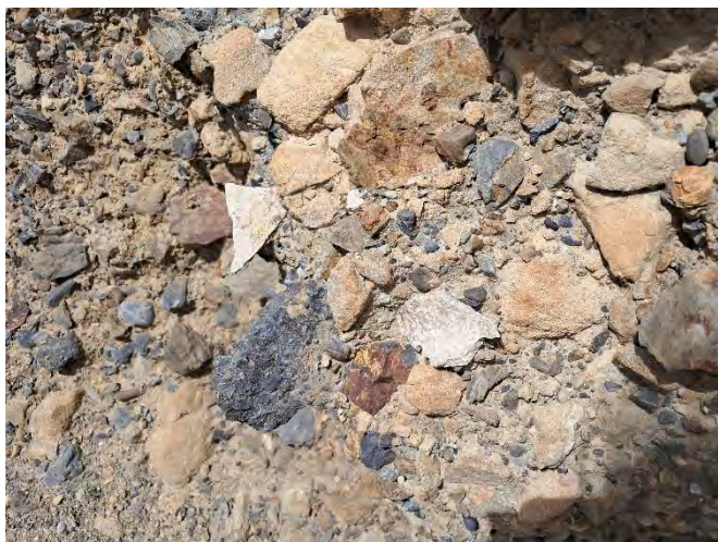
Photo 14. Suspected ACM and asphalt in exposed fill – within the eastern bank in line with 35 Moa Point Road.
