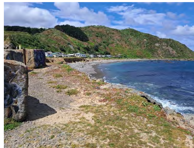
Photo 4. View from the seawall of the east area / eastern bank, facing south-east.
