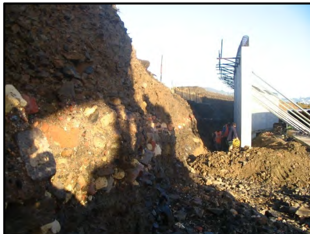
Figure 11. The soil profile on the south side of the tunnel
