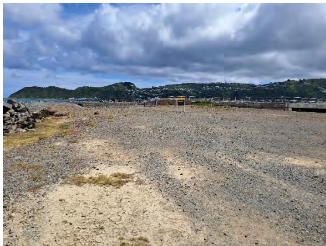
Photo 3. View of the seawall from the east side – other end of Moa Point Road tunnel visible far right.
