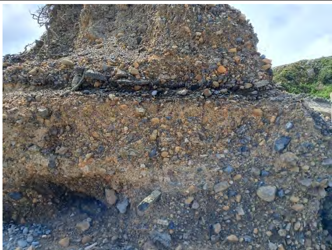
Photo 16. A portion of the exposed bank viewed from the beach – a layer of asphalt and timber is visible.
