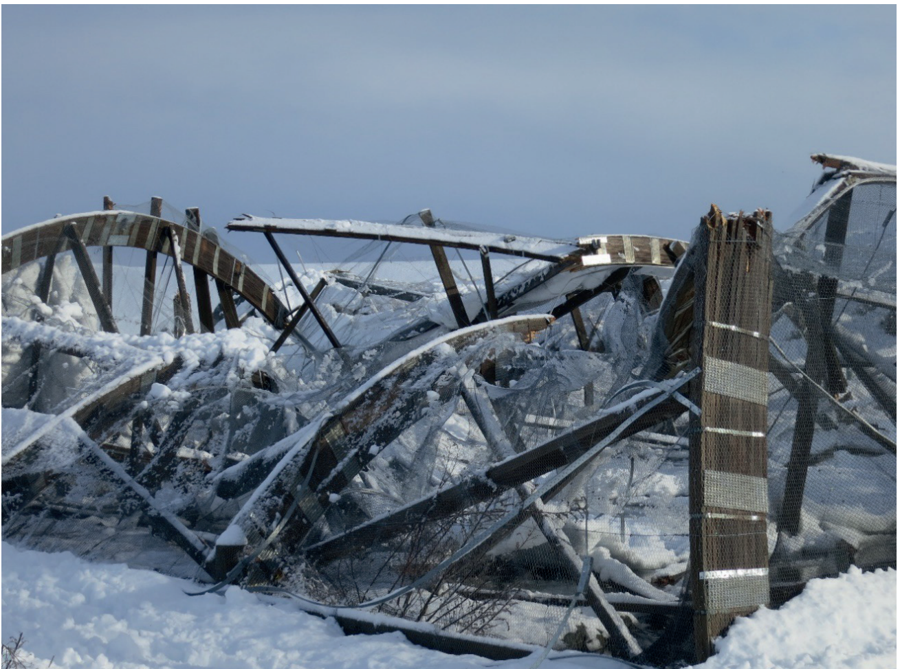
Aviary A collapse following heavy snowfall in 2015. Photo: Dean Nelson
