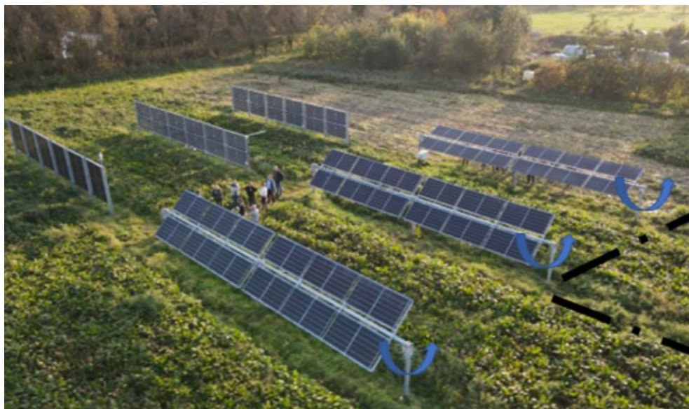
Figure 8. Examples of a solar farms demonstrating the use of vertical panels and creation of gaps among panel groups (From scientific paper by Willockx et al. 2023 -top and Krexner et al. 2024 - bottom)
