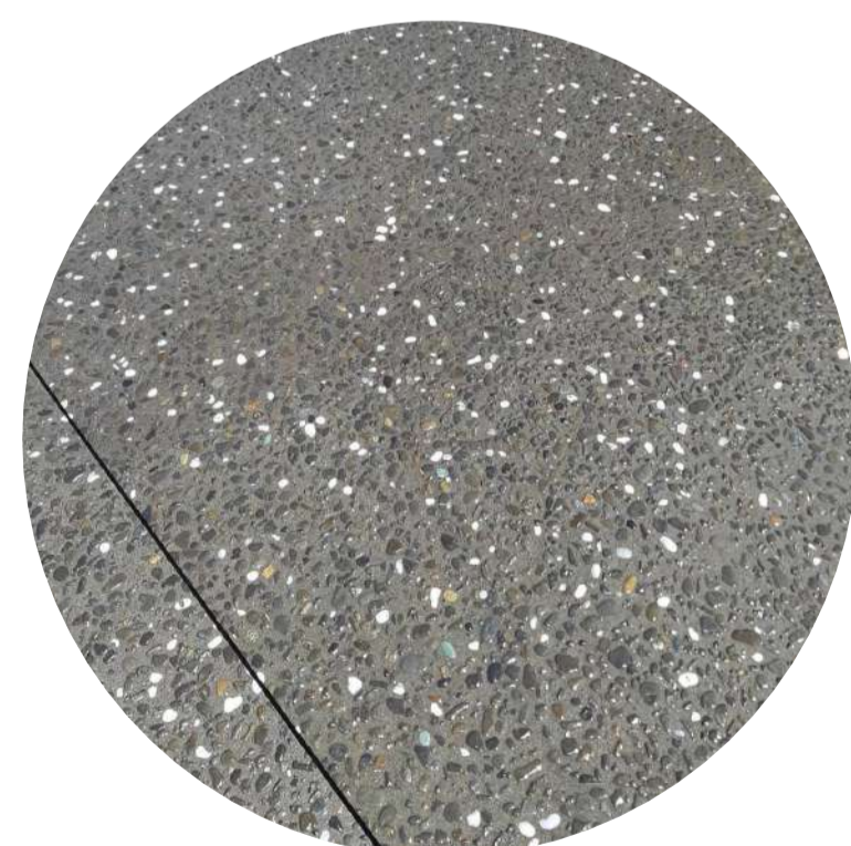
Exposed Concrete Driveway
