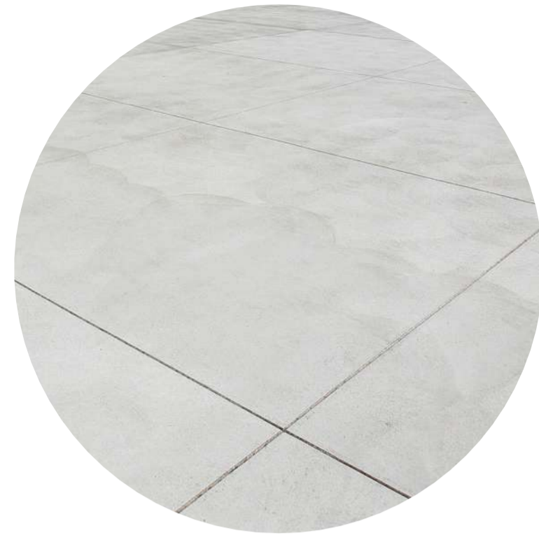
Concrete: Trowel Finish
