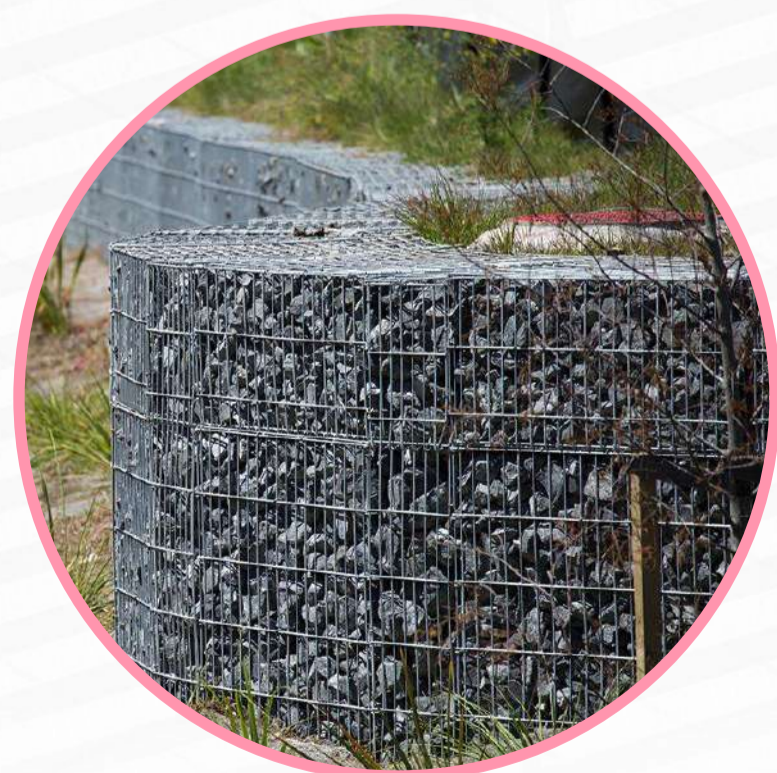
Low Gabion Feature Wall
