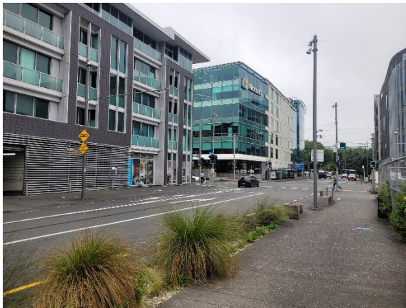
Figure 2.7 Sofitel and commercial office buildings across Halsey from the south-east corner of the site
