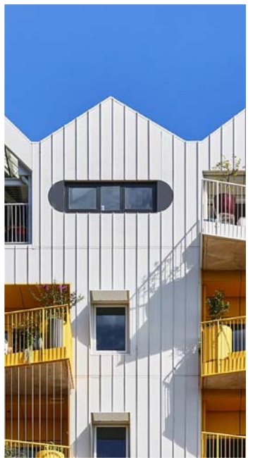
1 Metal cladding and roofing
