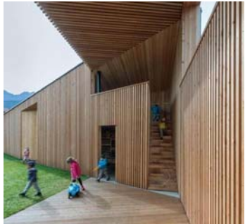
4 Stained timber cladding
