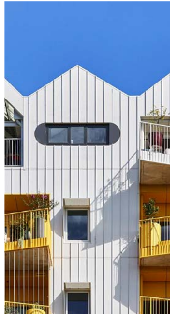
1 Metal cladding and roofing
