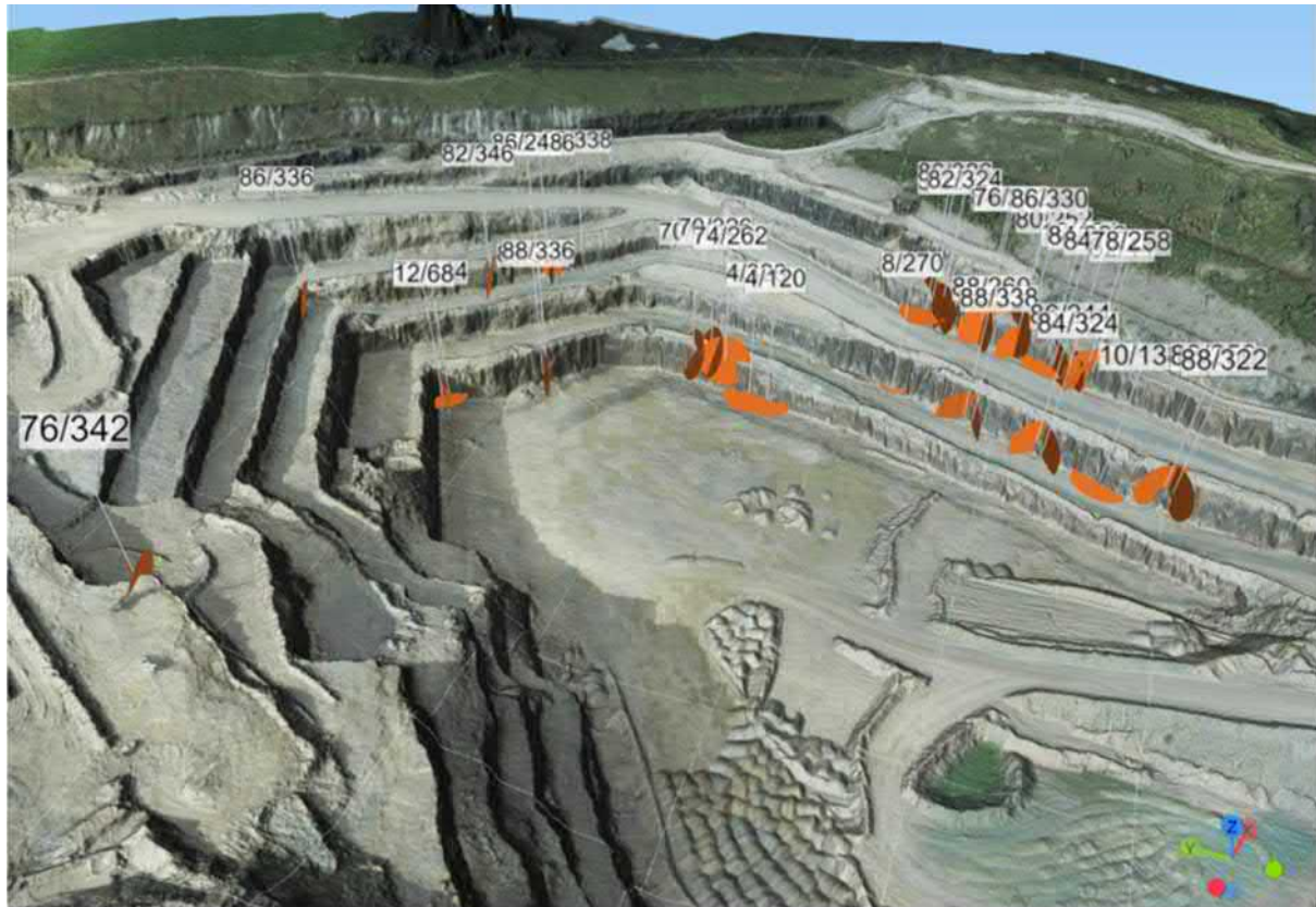
Figure 6-1: Observed structural defects [orange discs, labelled with defect orientation] within Oparure pit. Figure facing northeast.
