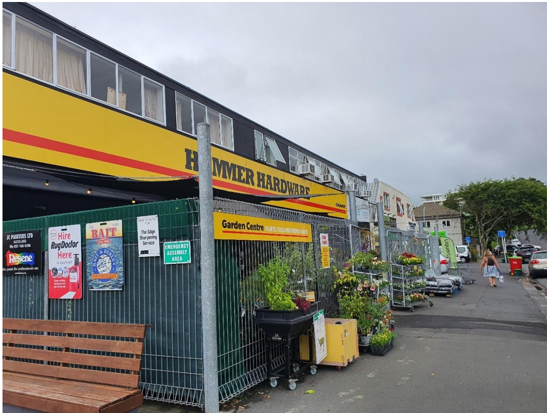
Photograph Appendix E.1: Looking southwest towards 15-21 Clarence Street.
