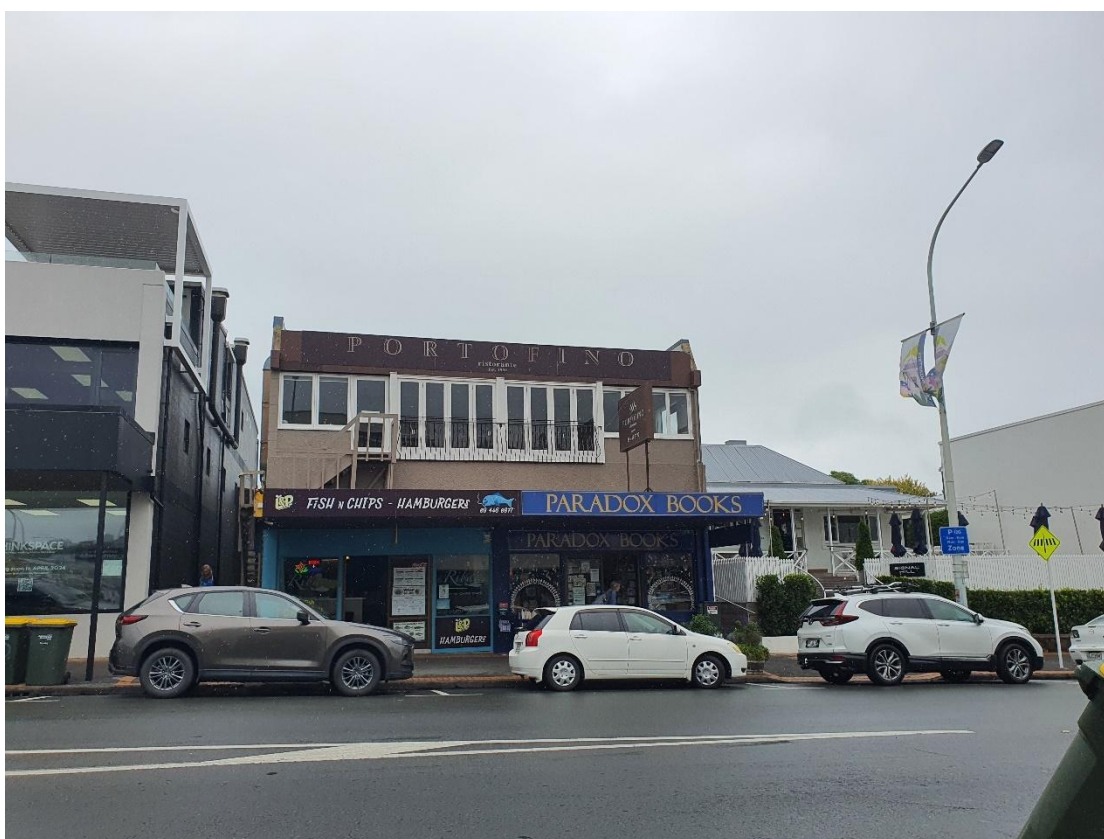
Photograph Appendix E.14: Looking east towards 24 Victoria Road.
