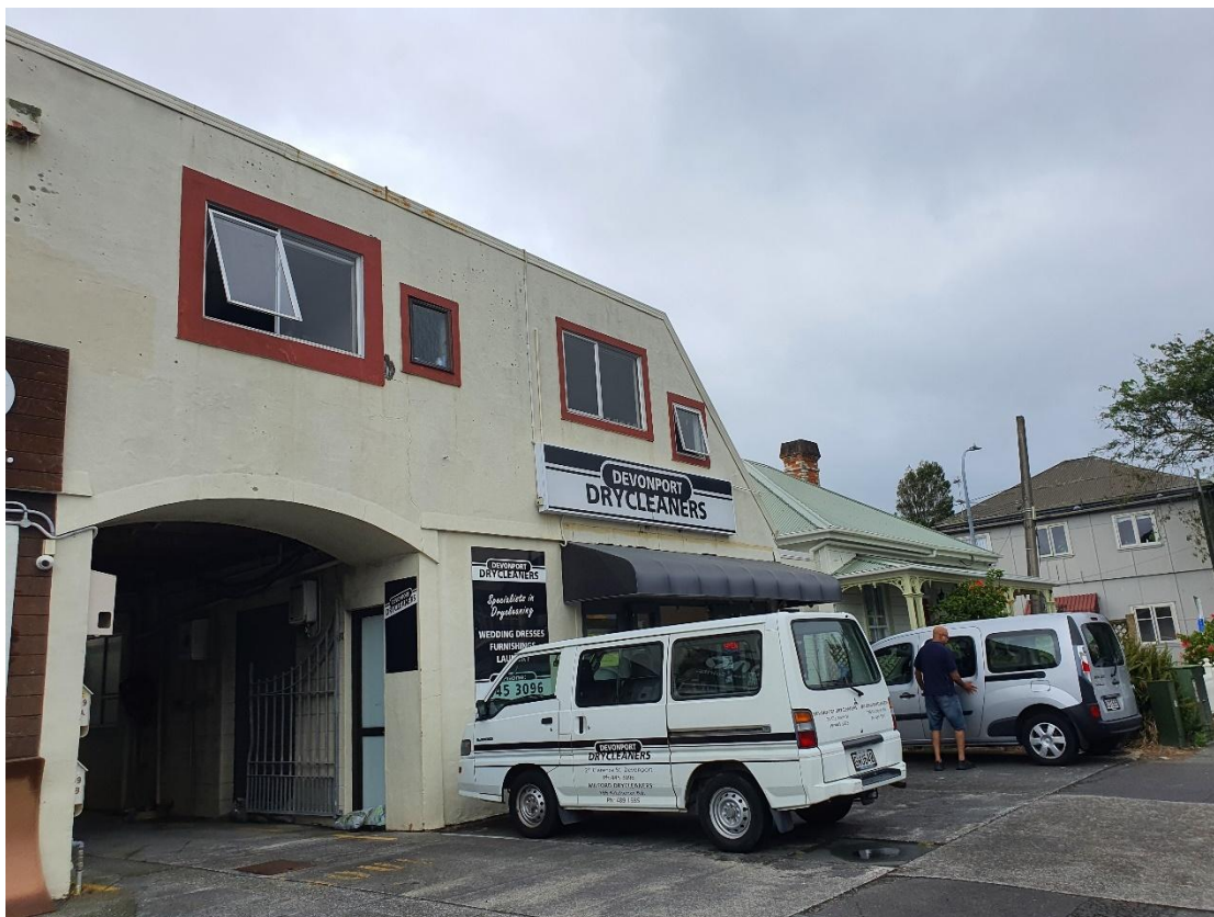
Photograph Appendix E.2: Looking southwest towards Devonport Drycleaners at 21 Clarence Street.
