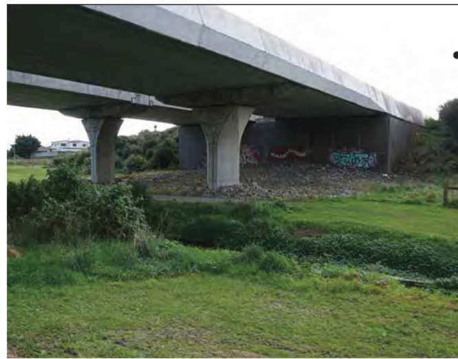
Expressway over Wharemauku Stream and footpath
