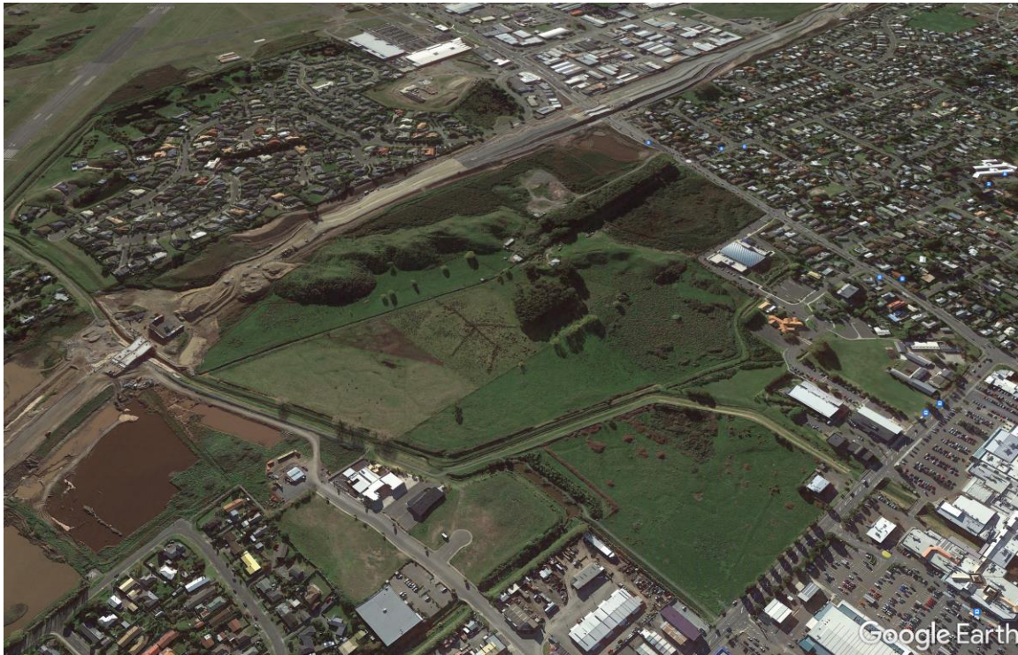
Figure 7: Google Earth aerial 2016. Shows M2PP under construction through the former dune ridge. Kapiti airport in the background upper left of frame and Paraparumu town centre bottom right.
