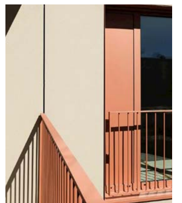
4 Feature recess cladding
