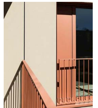
4 Feature recess cladding
