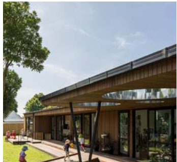
1 Large canopy, exposed structure
