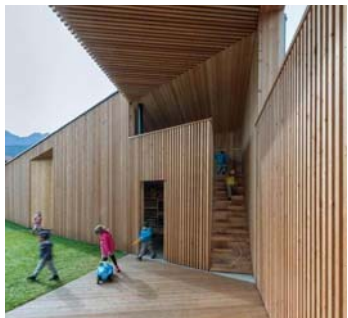
4 Stained timber cladding
