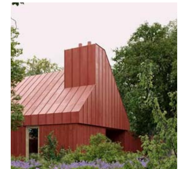
2 Metal wall and roof cladding
