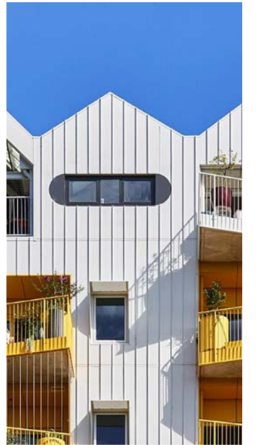
1 Metal cladding and roofing
