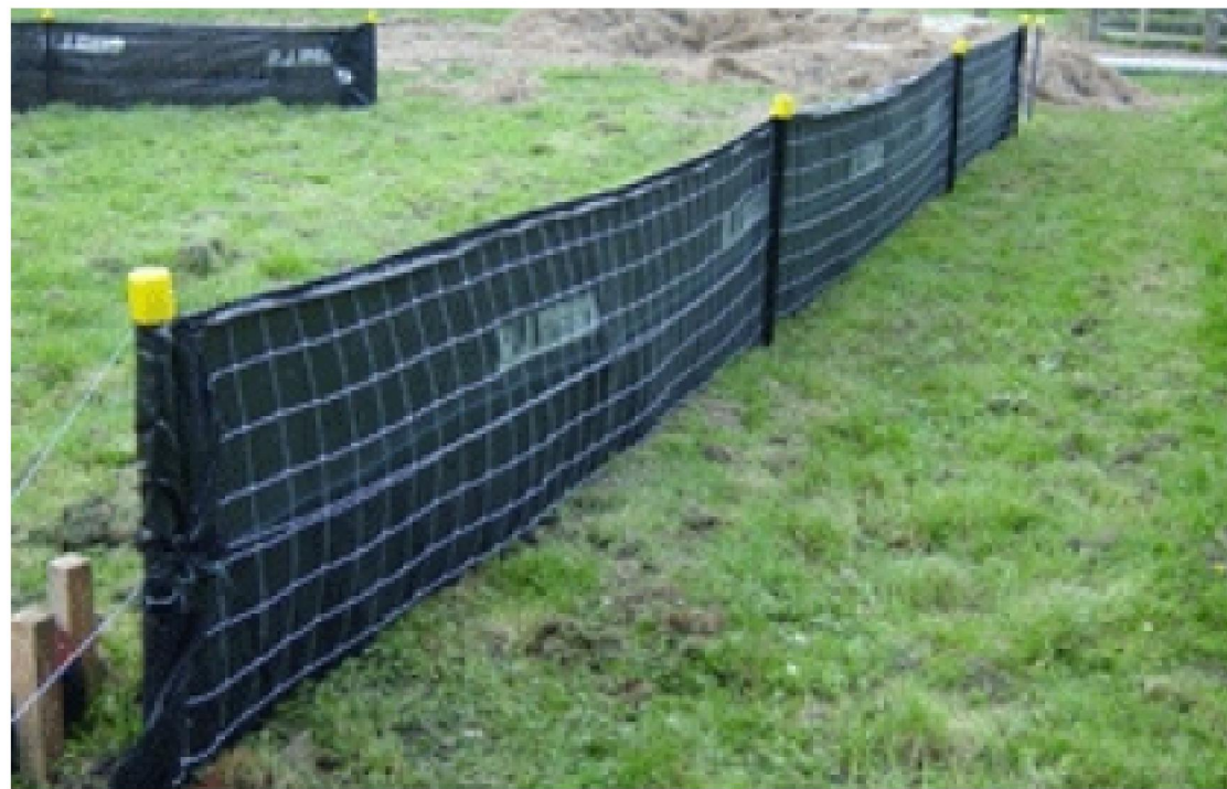
○ SUPER SILT FENCE CLOSE UP VIEW NOT TO SCALE
