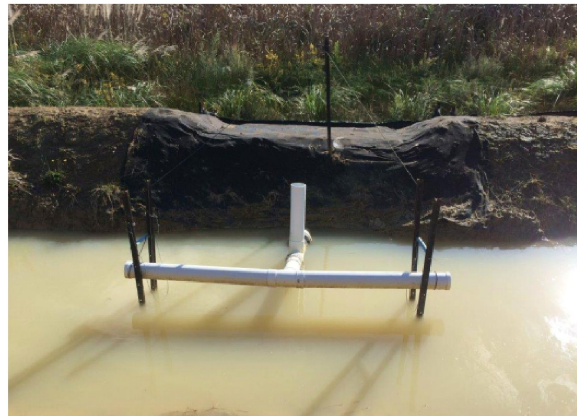
DECANTING EARTH BUND CLOSE UP VIEW
