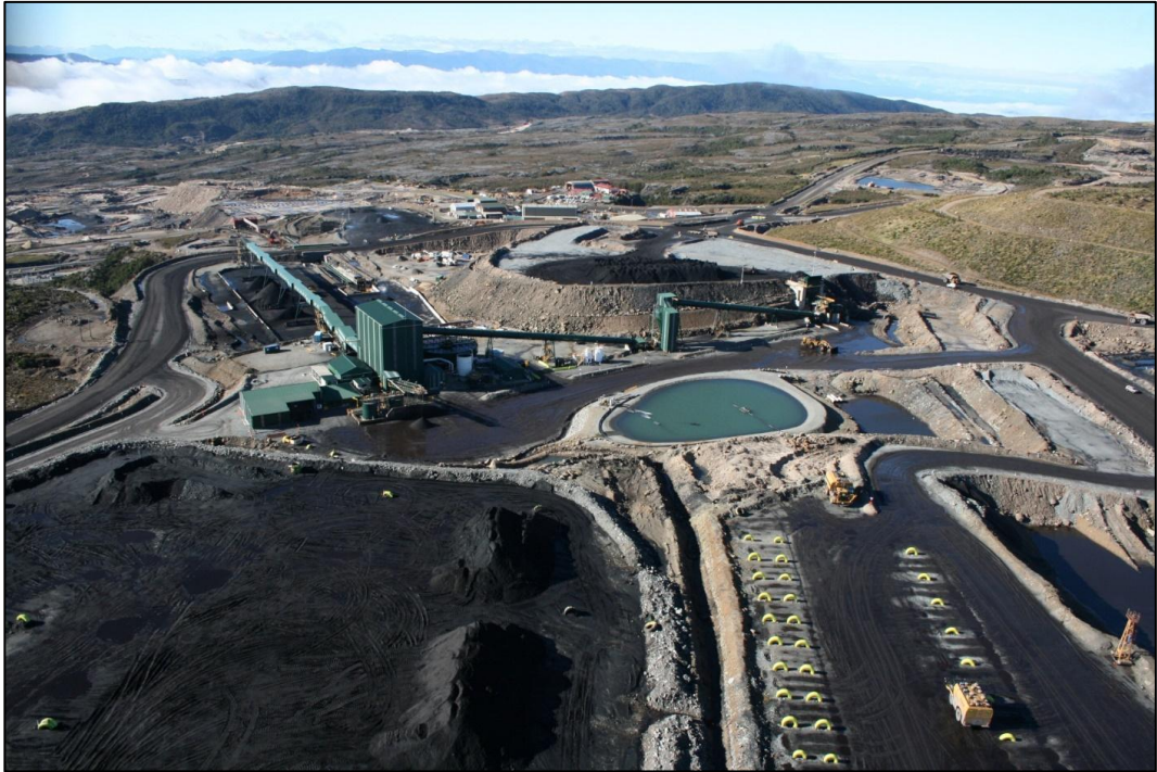
Figure 3-56: Stockton Coal Handling and Processing Plant Aerial
