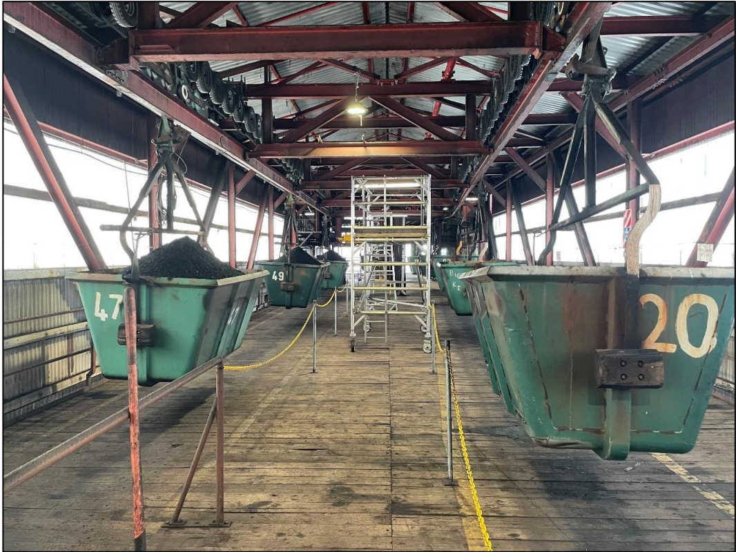
Figure 3-57: End of Aerial Ropeway at the Ngākawau Rail Loadout
