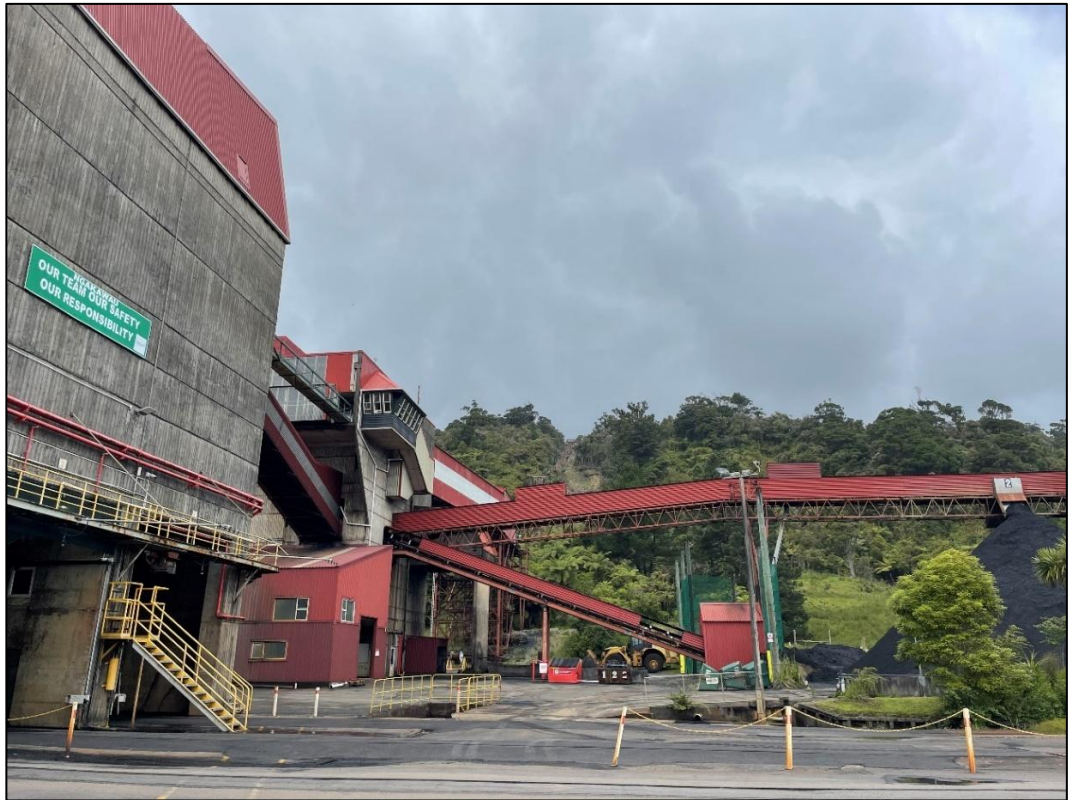
Figure 3-58: Ngākawau Rail Loadout
