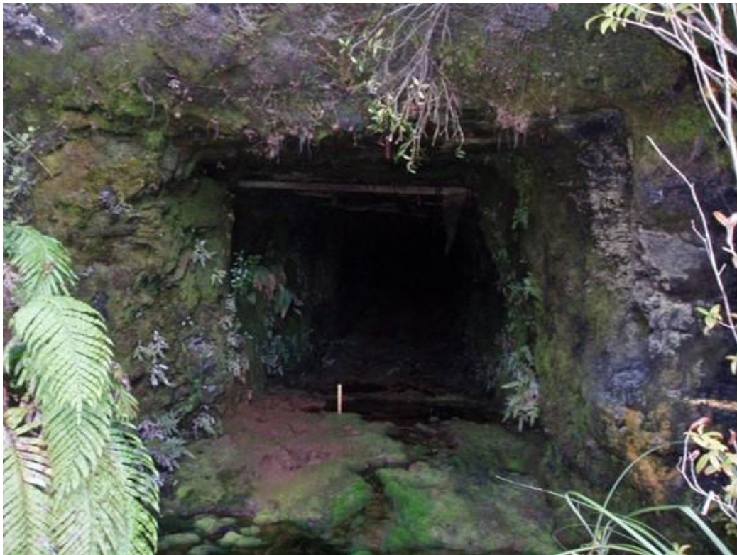
Figure 13. 'A' Tunnel portal (Waypoint 761) (Watson Jul 2008)
