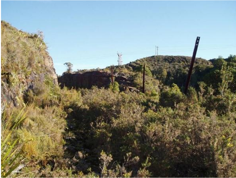
Figure 10. A cutting through rock on the Loco Line on the First Section. Note the power poles to the right and the aerial cableway in the distance (Watson Jul 2008)
