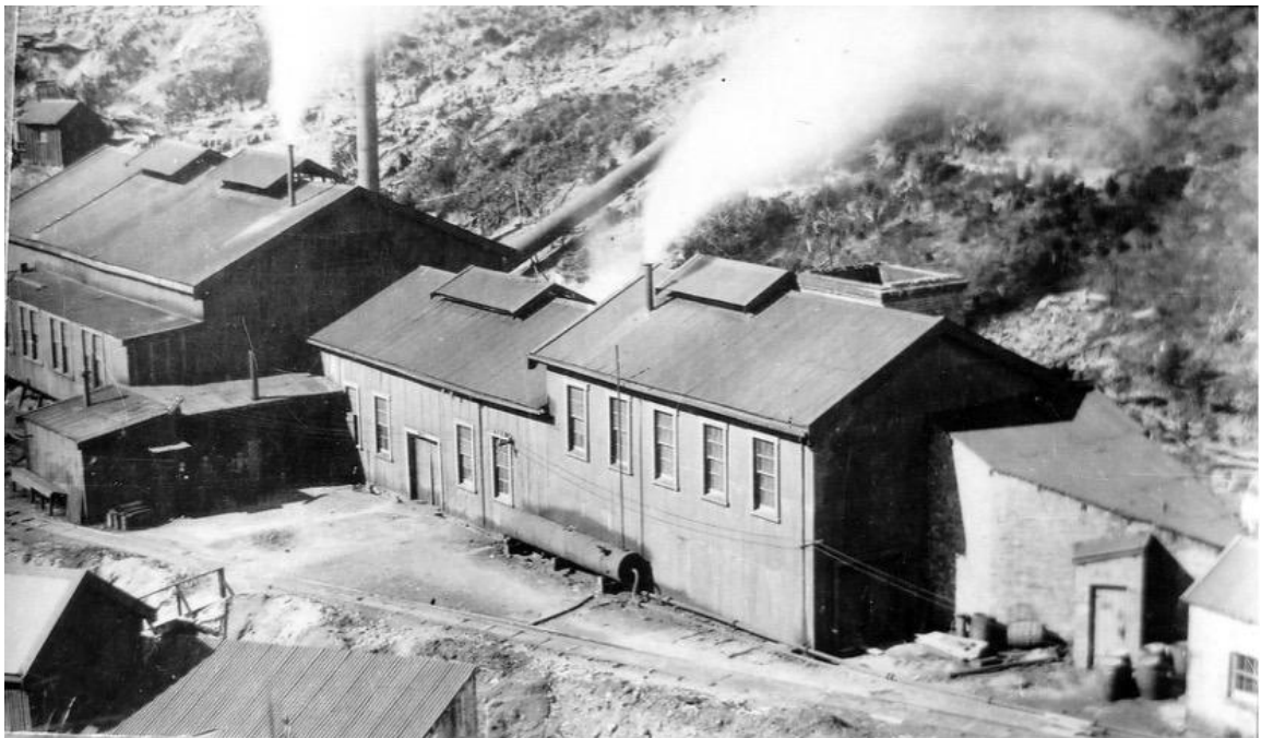
Figure 20. Boiler and air compressor sheds at Mine Creek (source: Coaltown Museum (Ref: MN56) in Watson 2007 Plate 9 Pg. 55)
