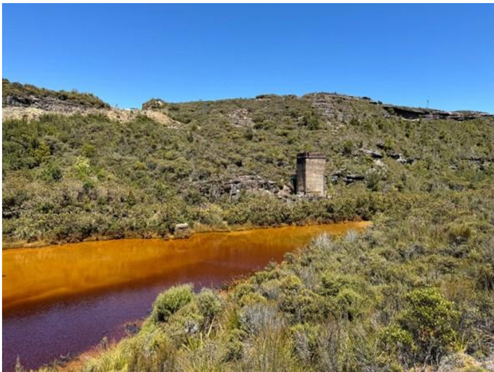
Figure 29. Looking south across the mine reservoir that encompasses Mine Creek to the brick ventilation flue and associated concrete foundations (wypt 101). The site of the air compressor and boiler sheds (wypts 52 and 53) is located on the terrace left of the brick flue (2024)
