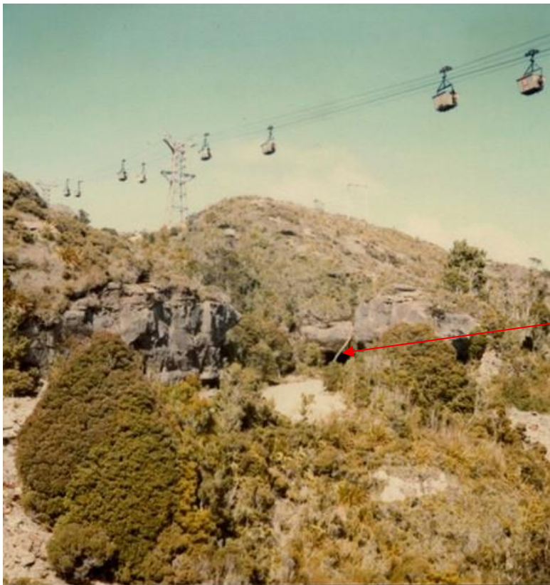
Figure 11. View from the Mine Creek Pack-Track of aerial cableway crossing the electric railway. 'A' tunnel entrance is in centre of photo (arrowed) (source: Sumner and Sumner 1983)
