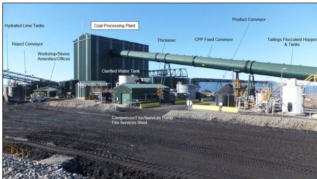
Figure 2.4: Coal handling and processing plant components (source: Bathurst).
