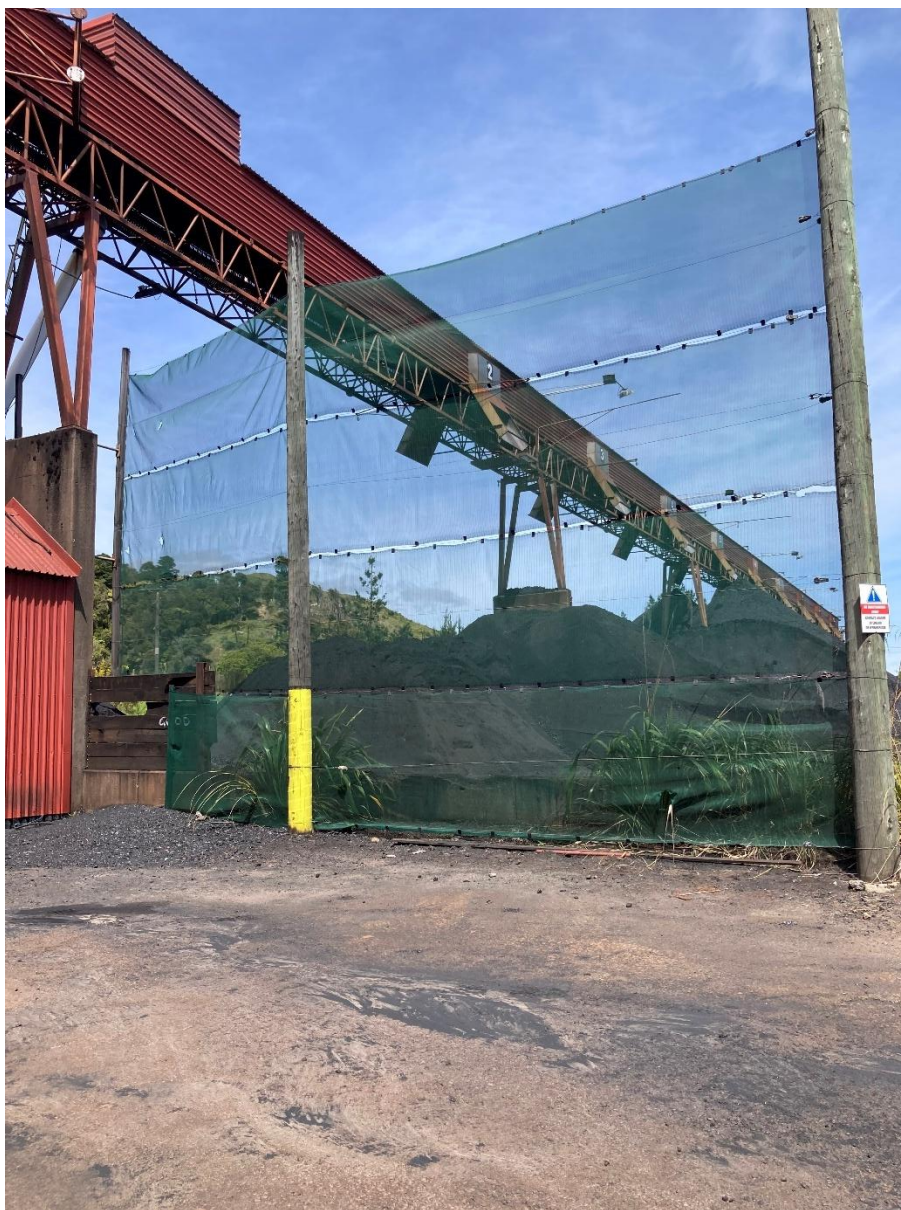
Figure 2.6: View of wind break fence.
