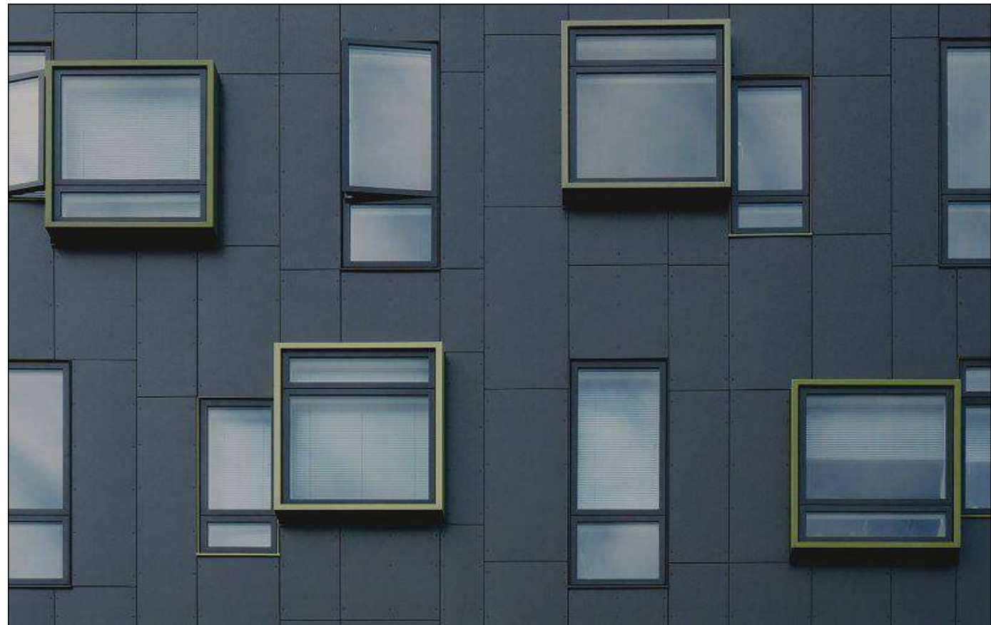
ACM - Facade panel (Rout & Return system)
