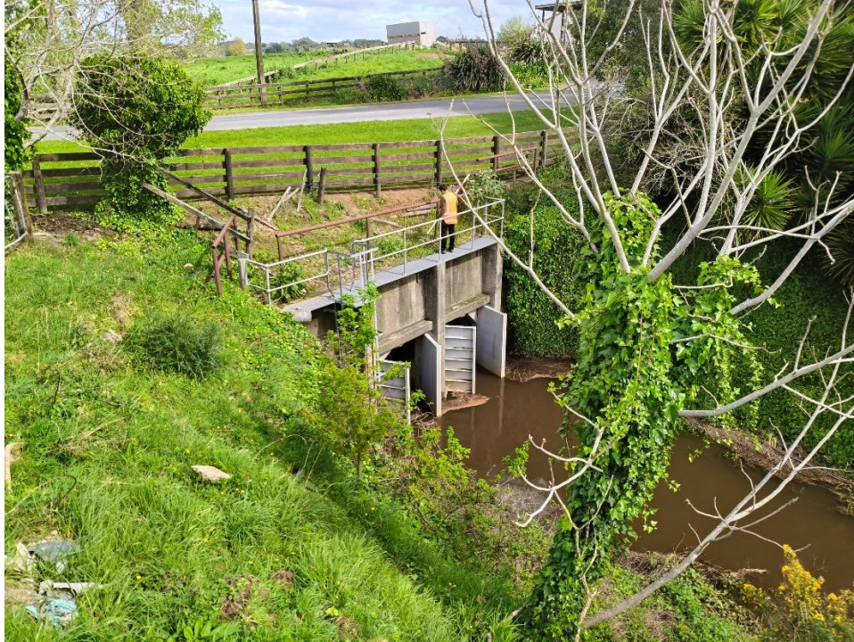
Figure 20: Existing Gate under Laxon Road.
