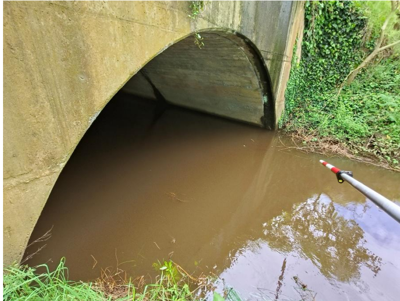
Figure 6: Laxon road culvert
