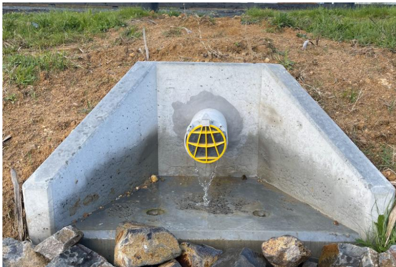
Figure 17: Backflow Device installed on Outlet Pipe.
