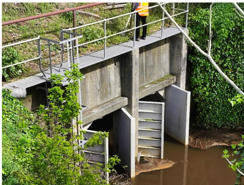
Figure 7: Culvert outlet with flood gates beneath Laxon road
