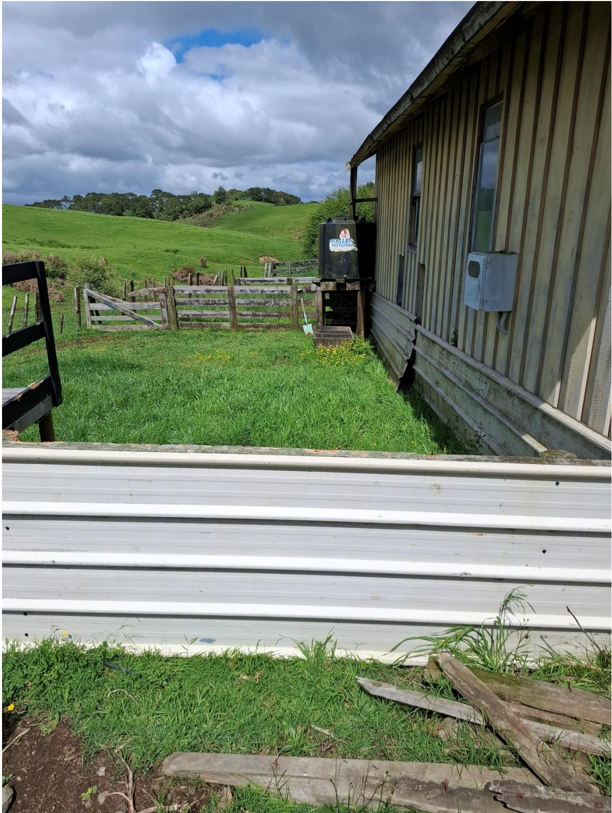
Figure 6: Building and Surrounds example.
