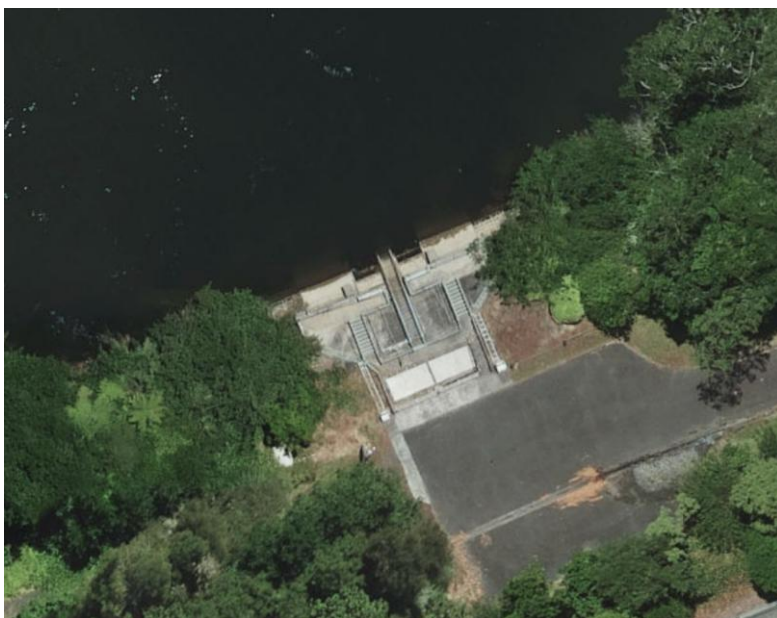
Figure 4: HCC intake on the Waikato River.
