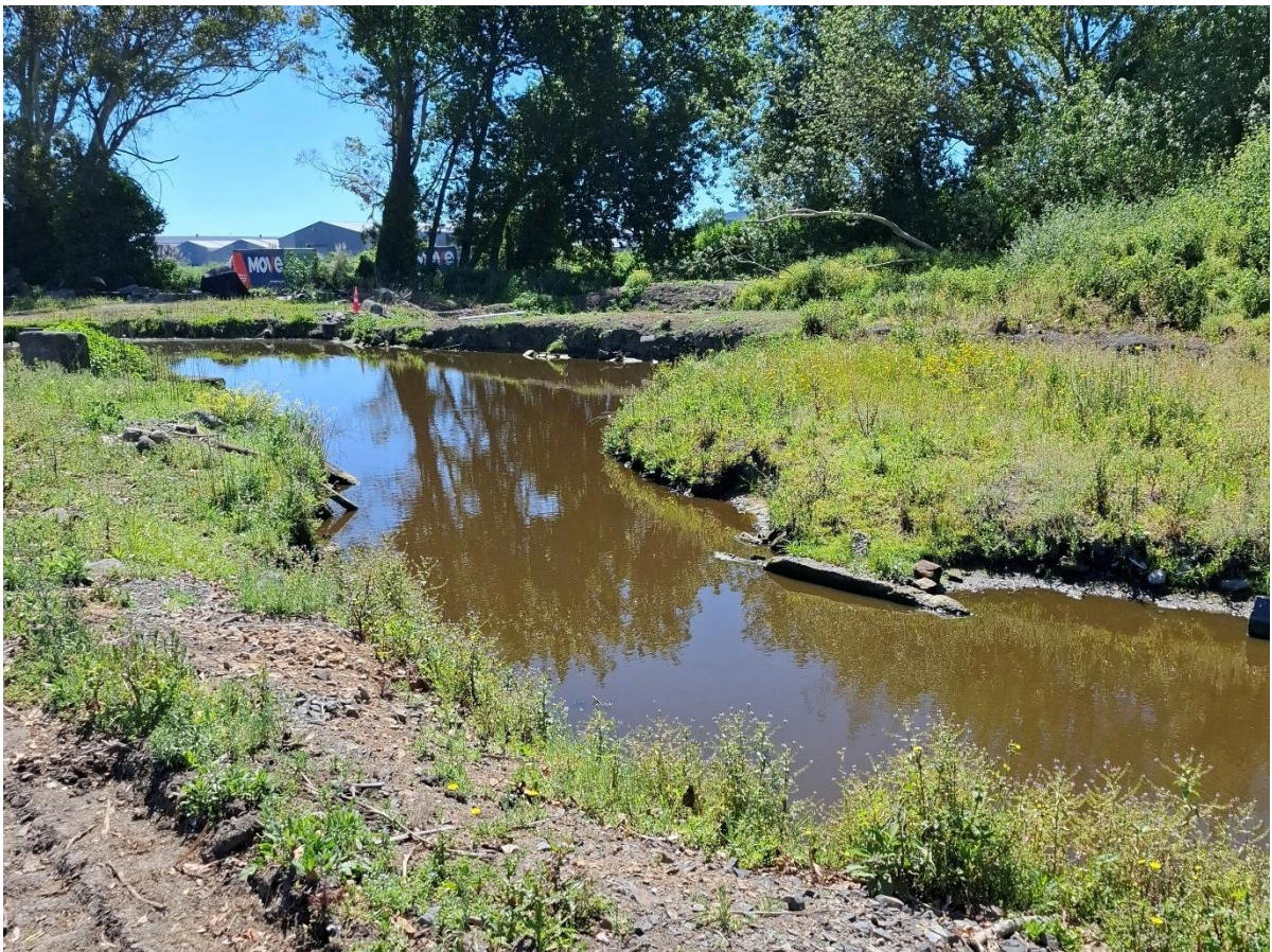
Figure 24: Artificial stormwater runoff pond within the EnviroNZ site.
