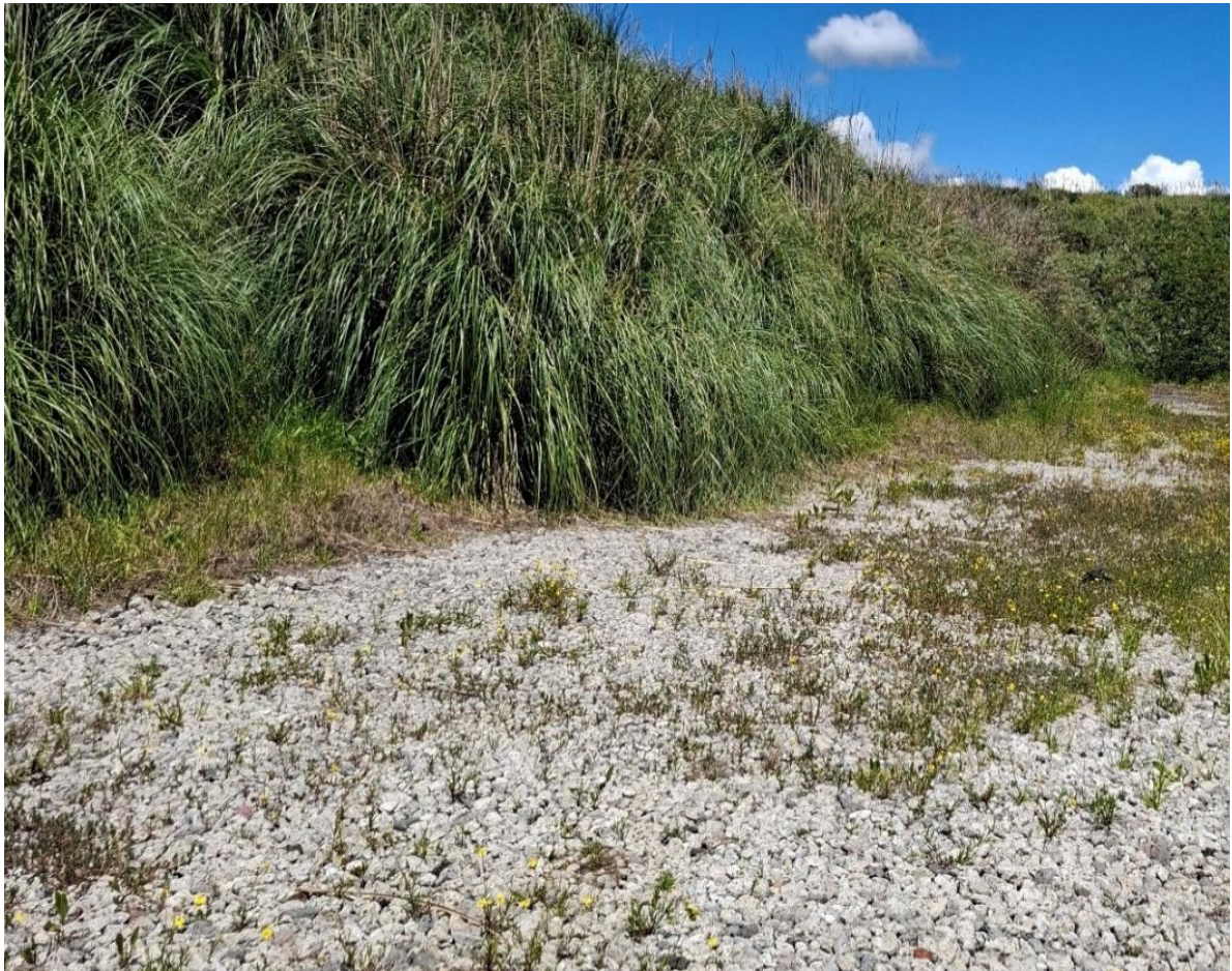
Figure 8: Loose rock track atop the cleanfill site and with dense pampas.
