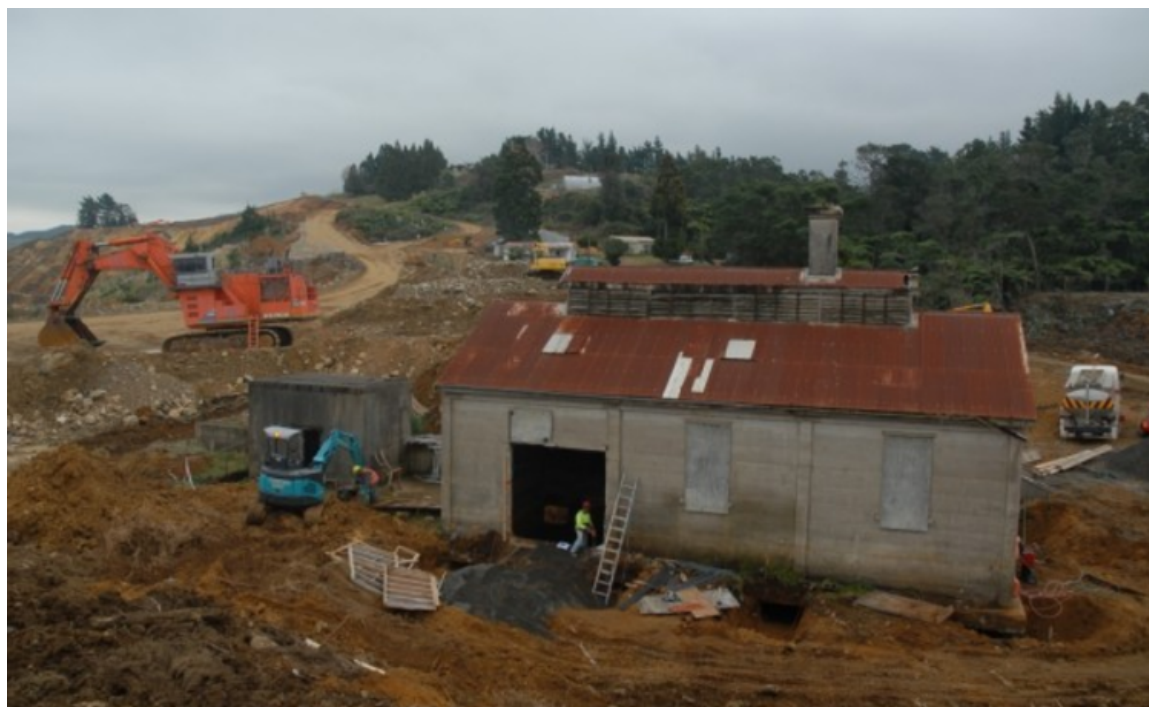
Figure 52. Grand Junction Refinery building and strong room being prepared for relocation in 2010 (source: http://www.waihigold.co.nz/about/history/grand-junction-refinery/grand-junction-refinery-building-on-the-move-in-2010/ )
