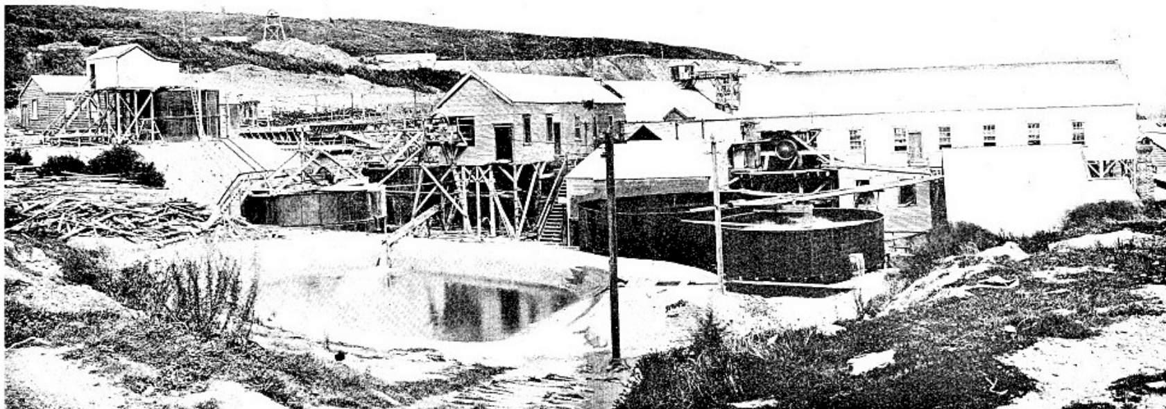
Face p. 85.] General View of Waihi Gold mining Company's 90-stamp Mill and Cyanide Plant at Waihi: Battery-water Reservoir, Settlers, Press Buildings, Agitators, and Solution Tanks in the foreground C.—3.
