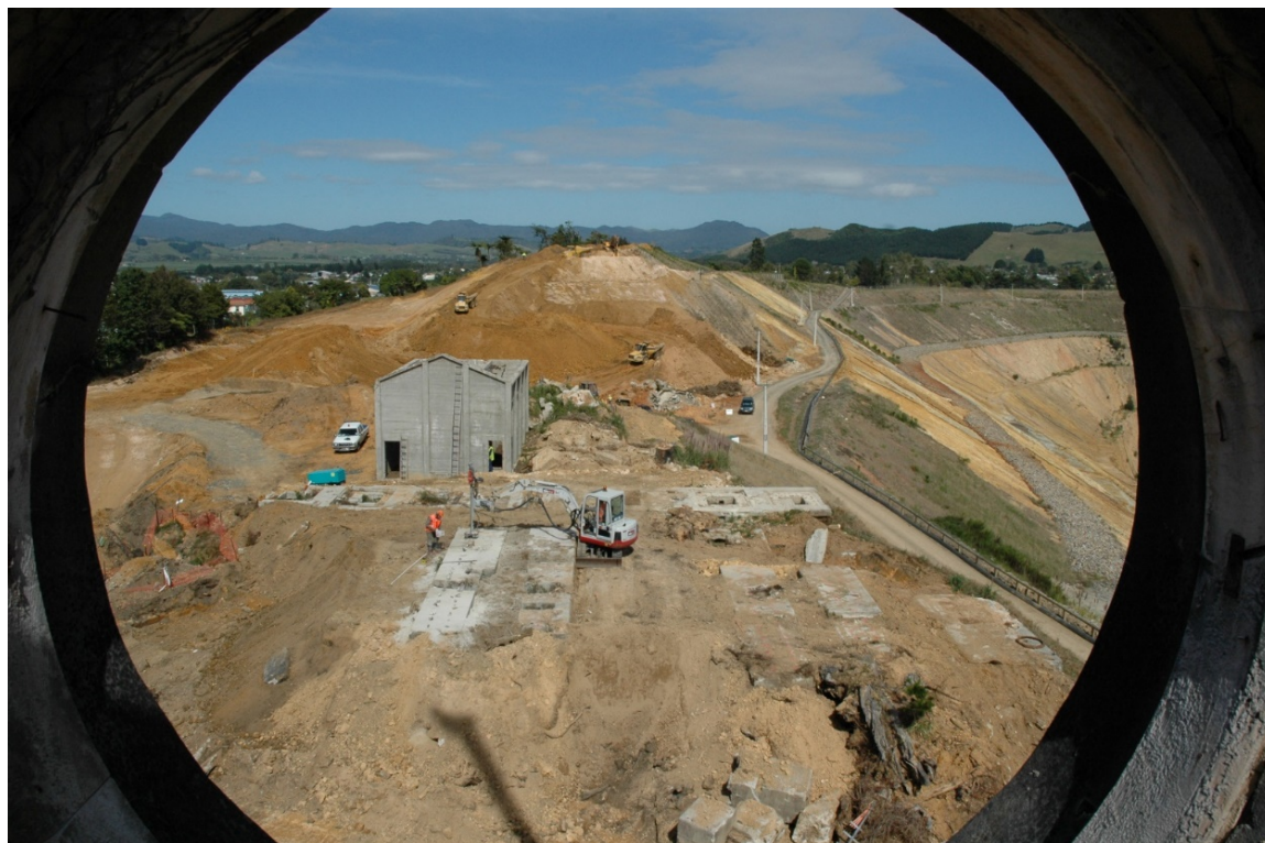
Figure 51. View west of transformer house prior to demolition from top of pumphouse (in original location), gas engine foundations and compressor pads (being drilled for explosives) this side of transformer house (source: Newmont Waihi Gold photo: 2006)
