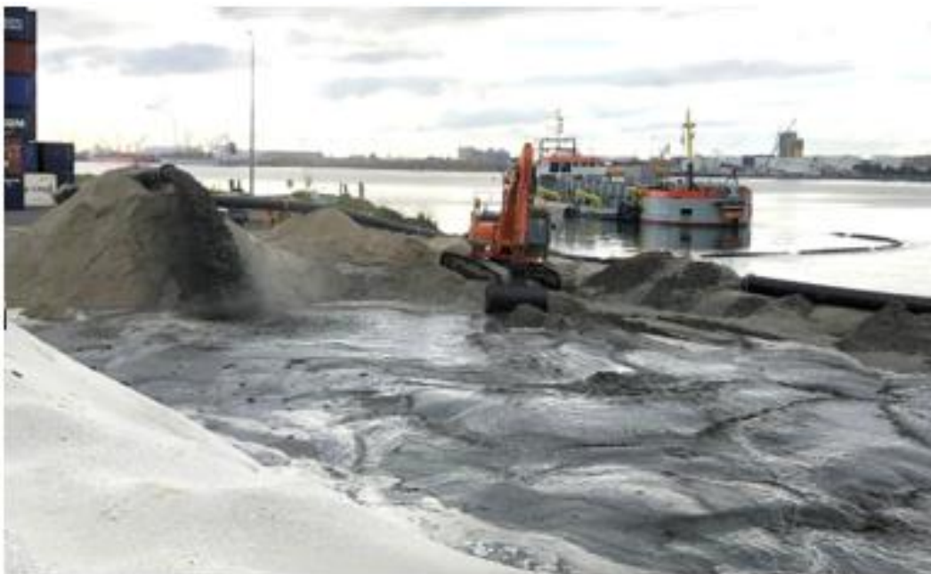
Plate 1: Pumping of dredged sand into the sand pile site. June 2019. Image supplied by POT.
