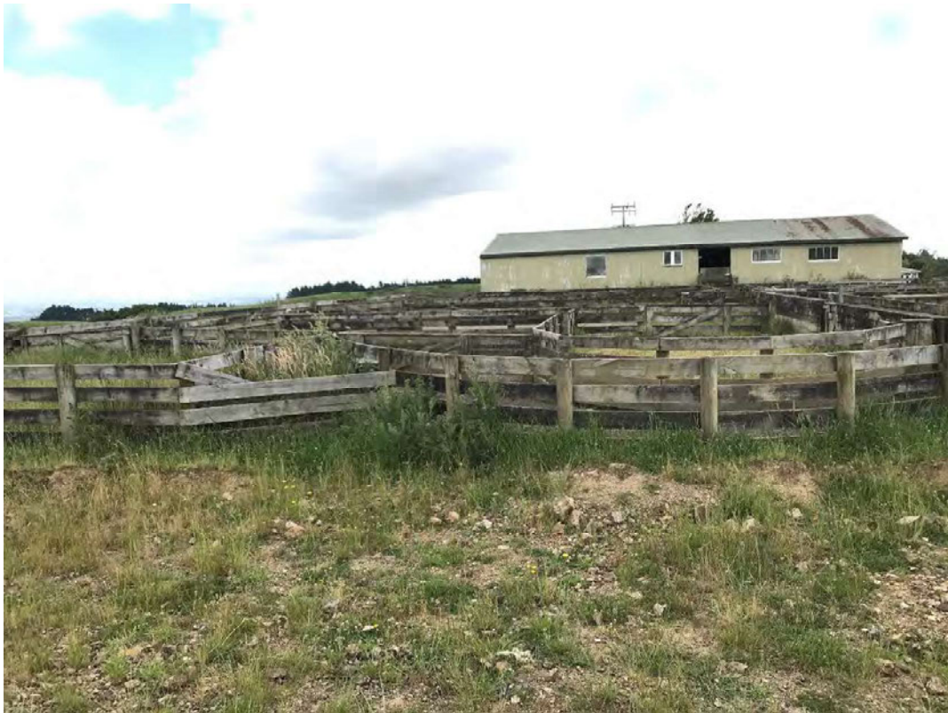
Photograph 4: Looking west at the potential location of the former spray race/sheep dip structure with the shearing shed in the background.
