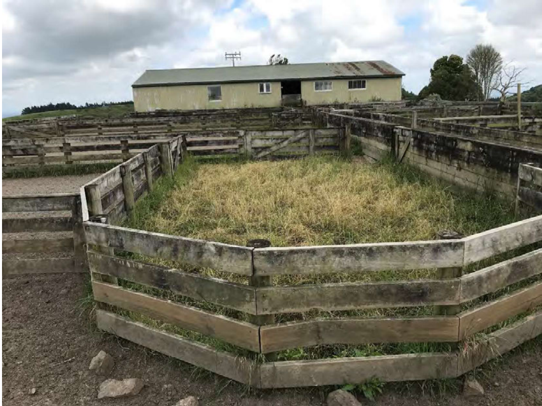
Photograph 5: Stressed grass within the potential location of the former spray race/sheep dip structure.
