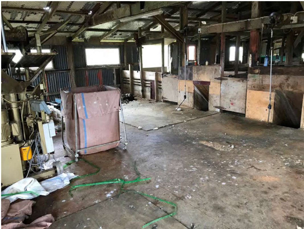
Photograph 7: Interior of the shearing shed.
