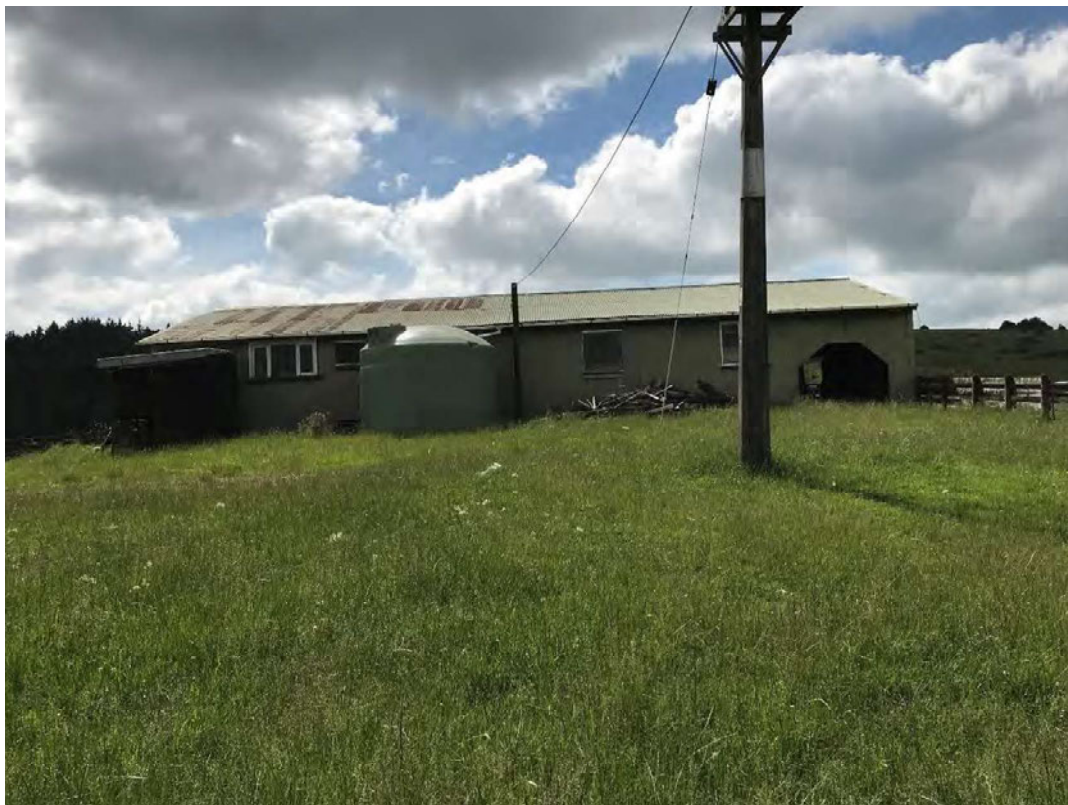
Photograph 6: Looking east at the shearing shed.
