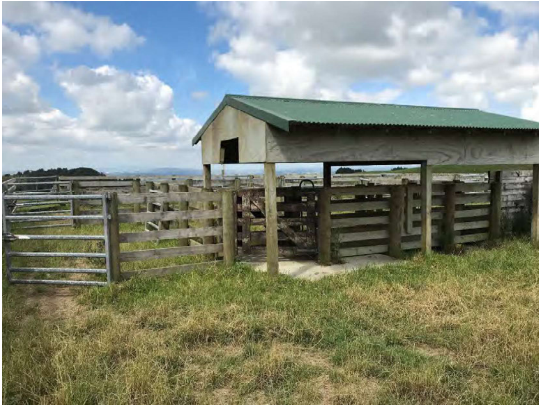
Photograph 13: Looking south at the potential location of the former spray race/sheep dip structure.
