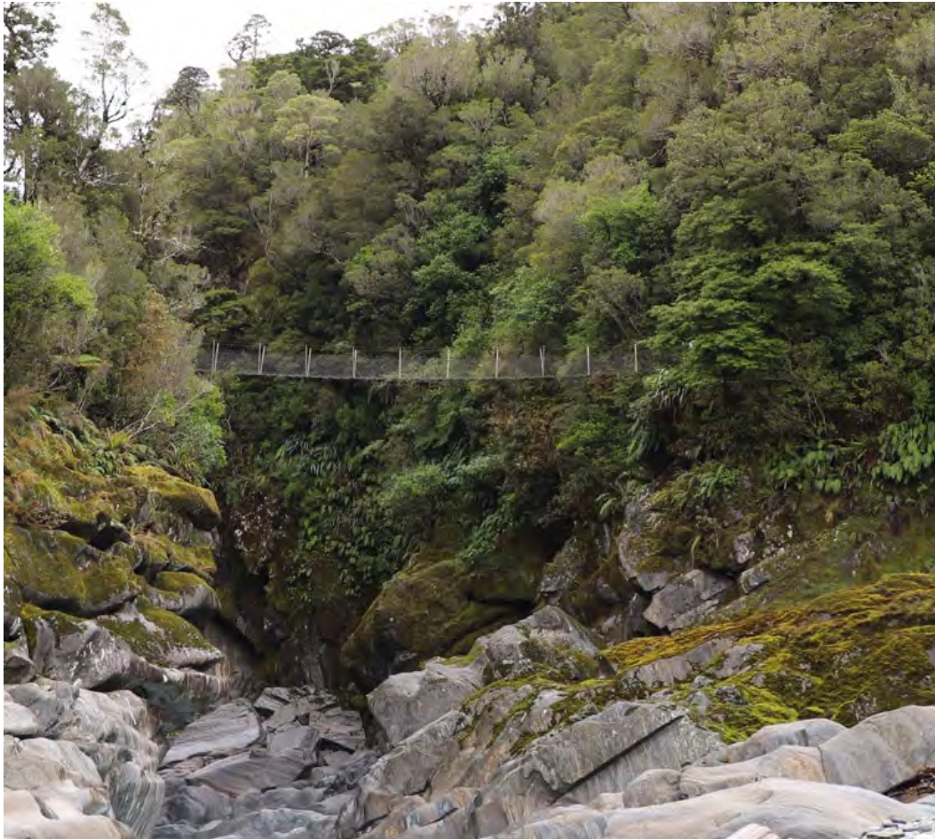
Figure 27: Photo of the swing bridge near the head of the Morgan Gorge
