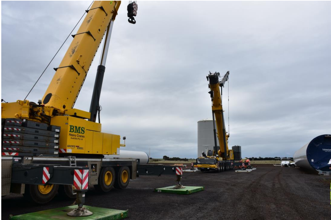
Figure 4: Photo of a wind turbine platform area, with cranes to assist with the wind turbine installation.
