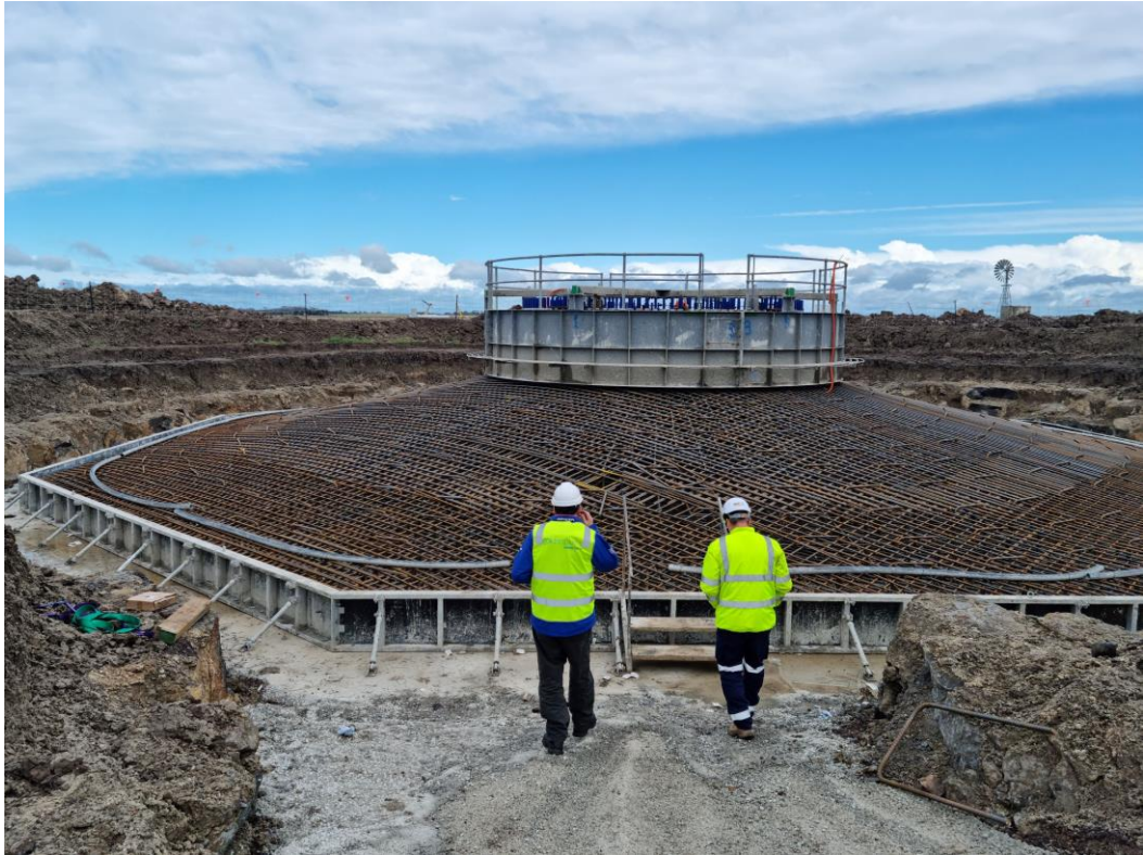
Figure 3: Photo of a wind turbine foundation during construction.
