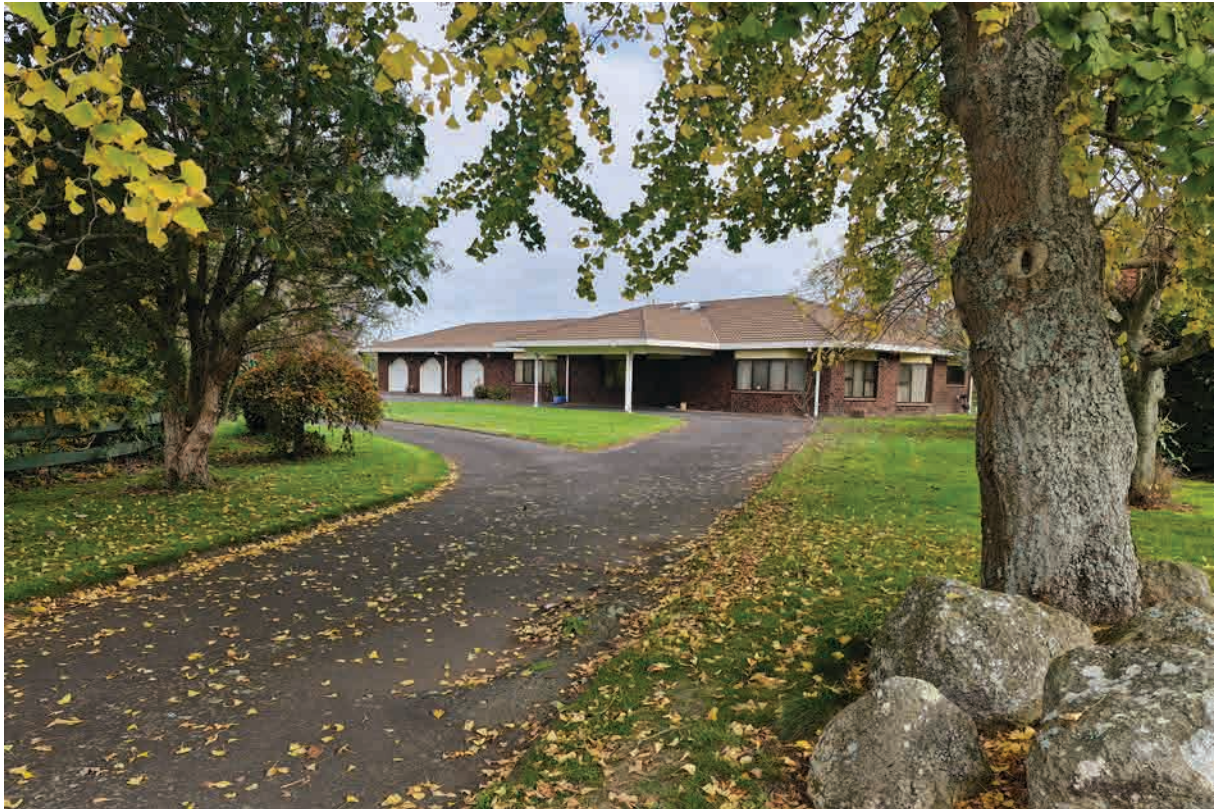
Figure 7. View of the east end of the property and house facing southeast.
