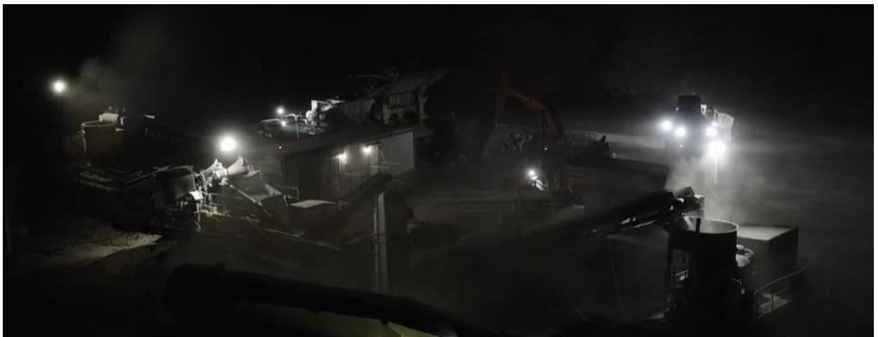
Figure 2. Typical mobile construction site lighting
