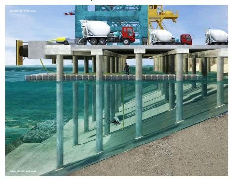
Figure 3 Concrete Mattress Installation (from Proserve)
