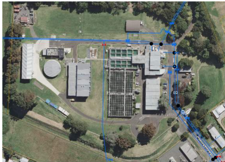
Figure 11: HCC Water Treatment Plant
