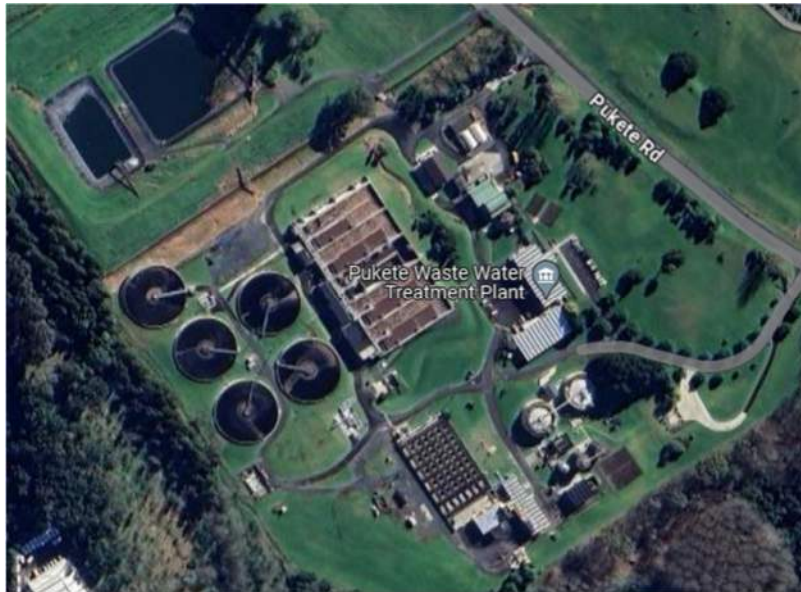
Figure 6: Pukete Wastewater Treatment Plant (Google Map)
