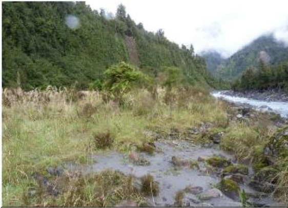
Photograph 10: The proposed powerhouse site near river level with the 60-70m high terrace edge in the background.
