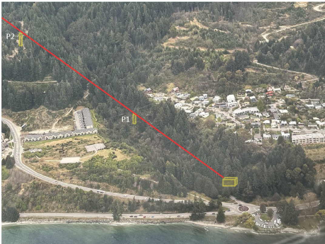
Photo 4: Approximate alignment of lower gondola route from One Mile Powerhouse Reserve station via pylons 1 & 2.
