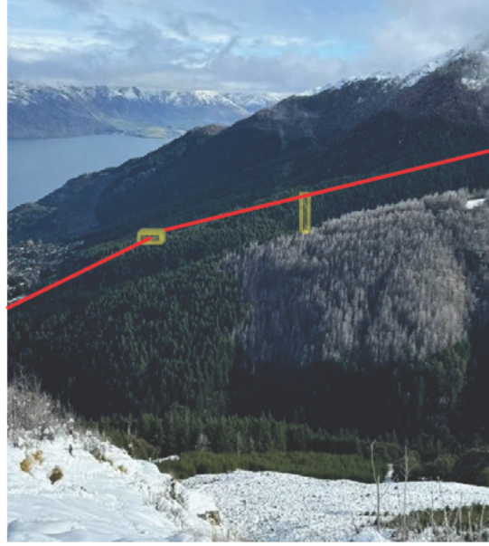
Photo 6: Fernhill Heights Station to rear and Pylon 3 on ridge between One Mile and Two Mile Creeks.
