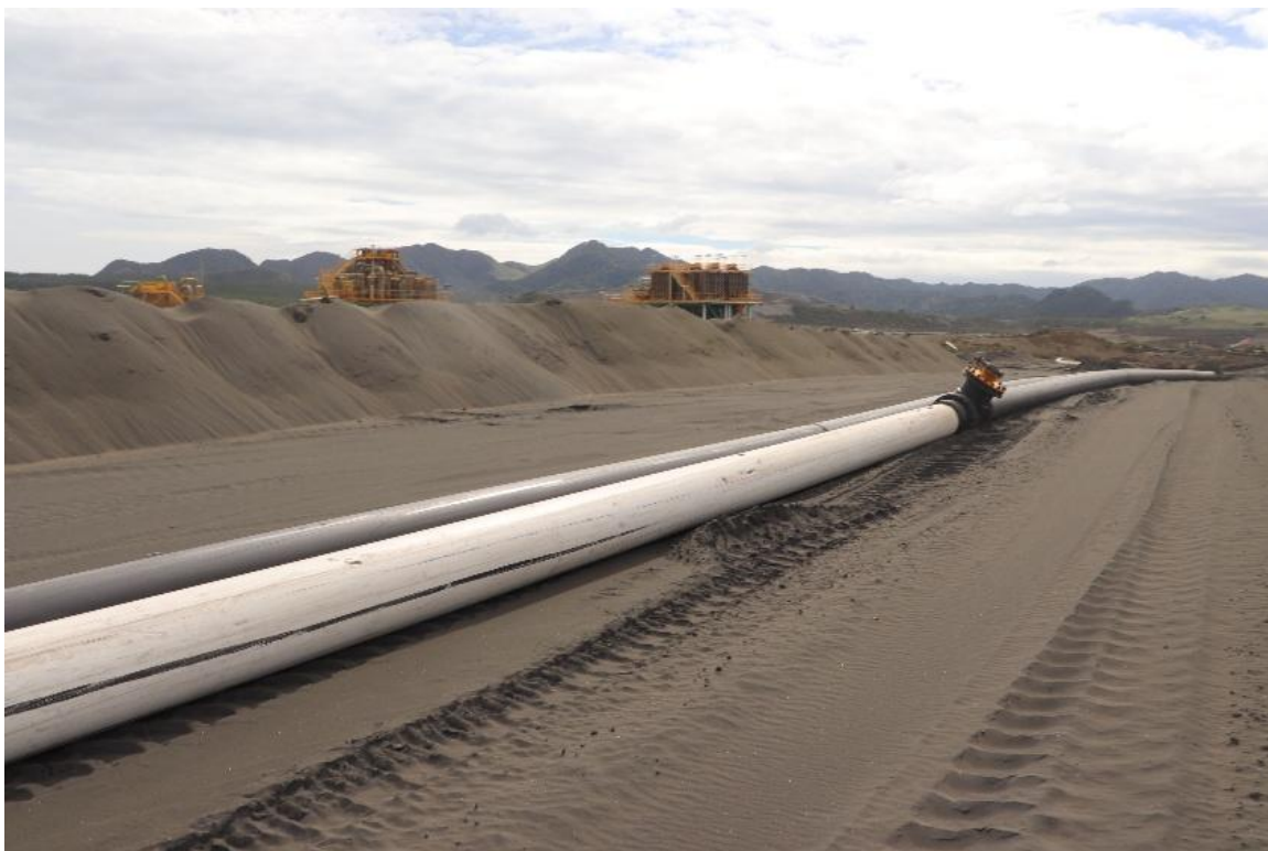
Figure 40. View southeast over recorded location of R16/68
