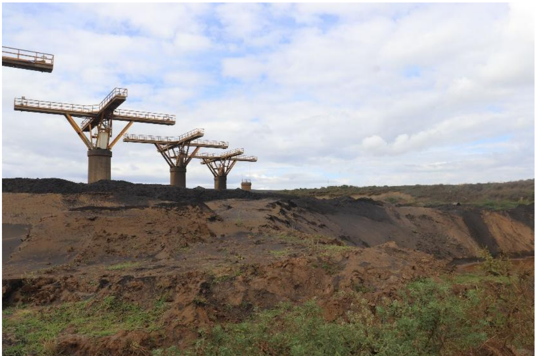
Figure 88. View southeast over recorded location of R16/213
