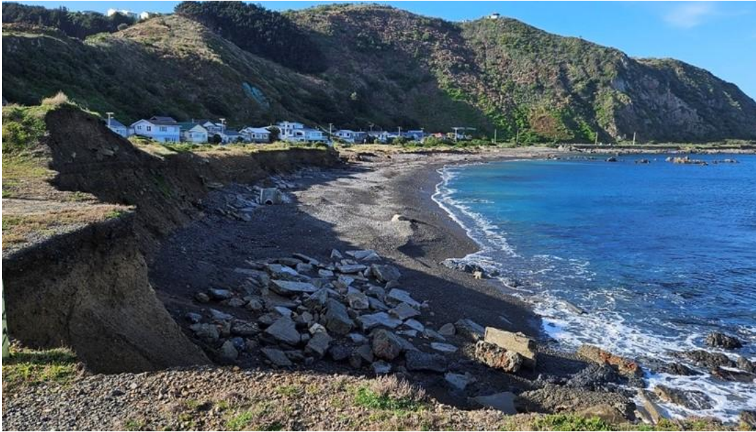
Fig. 4.8. View of the eroding earth bank (Construction Area F), looking eastwards from the eastern end of the informal seawall.
