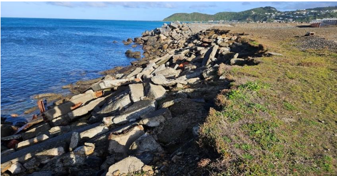
Fig. 4.6. View of the informal eastern area seawall (Construction Area D), looking westward towards the Southern Seawall.
