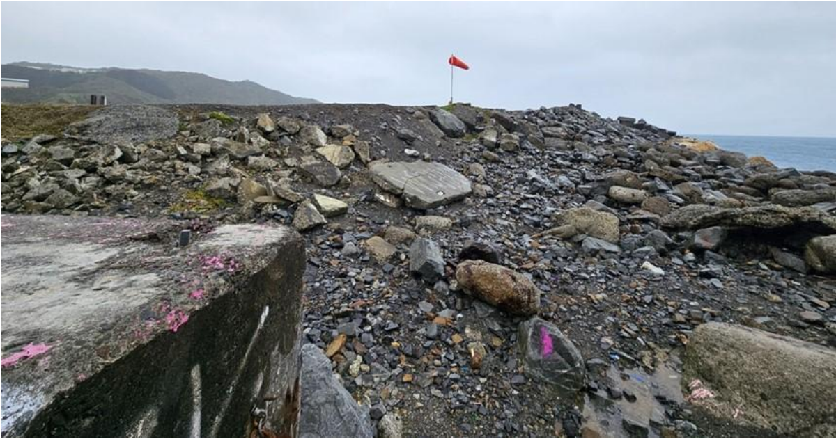
Fig. 4.5. View of construction area A, looking southwards.
