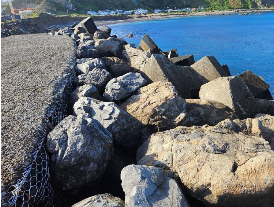
Fig. 4.7. View of the eastern end of the Southern Seawall (Construction Area C), looking eastwards.
