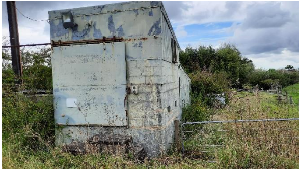
Photograph 3: Livestock farm structure
