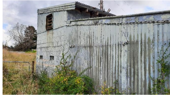
Photograph 4: Southern side of the livestock farm structure
