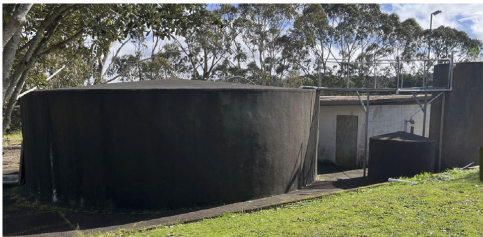
Figure 48. Photograph showing the water tank beside the community hall, looking northwest
