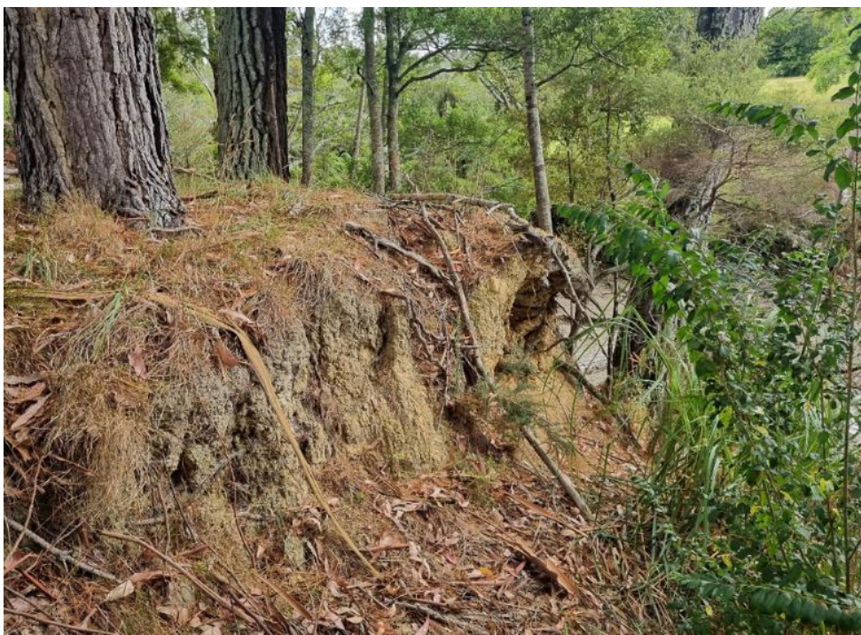
Figure 32. Photograph showing exposed section of eroded creek bank in Area 2
