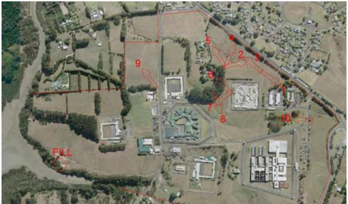
Figure 20. Aerial plan showing the areas that were photographed during the 2013 survey (source: Felgate 2013:16)
