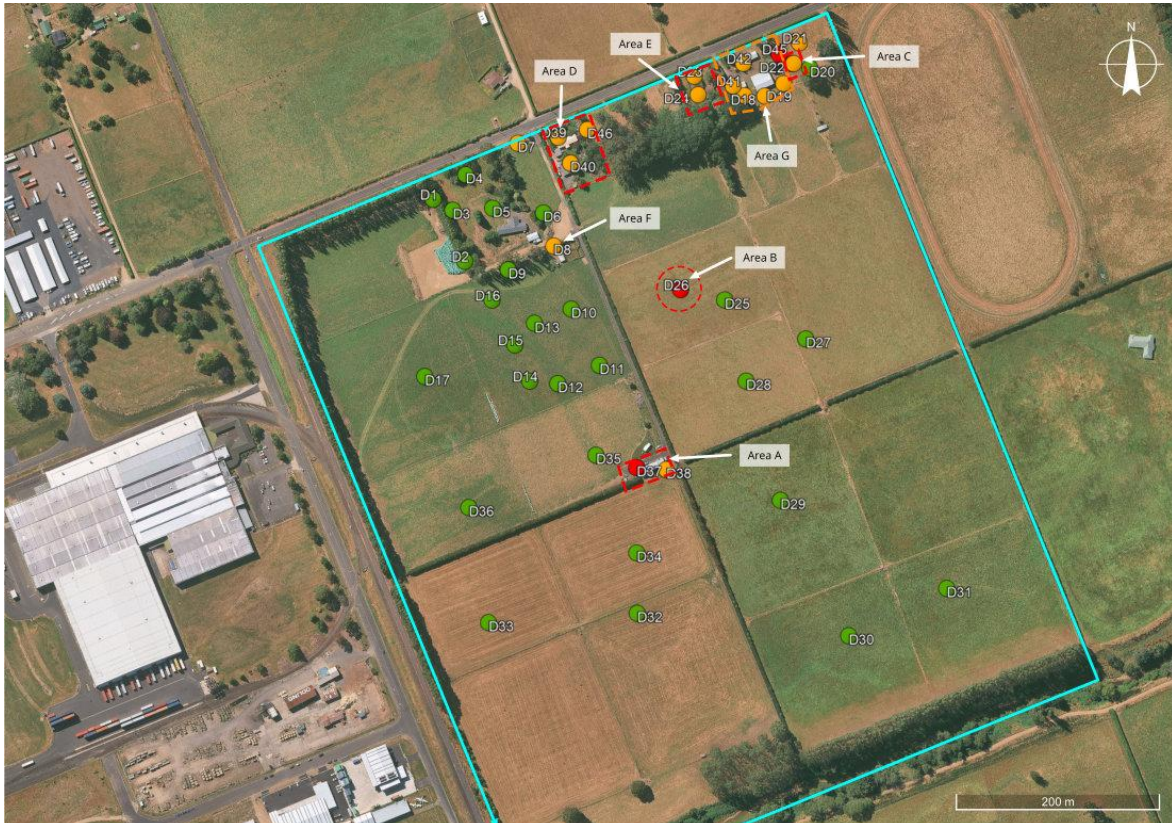
Figure 6: Sampling locations from the DSI. Red indicates samples that exceed the Commercial/Industrial SCS/SGV, and orange indicates samples above background but below the Commercial/Industrial SCS/SGV. Green indicates samples consistent with predicted background. Areas outlined in red indicate verified HAIL sites and areas outlined in orange indicate unverified HAIL sites (Google Earth, Image © 2025 Airbus).
