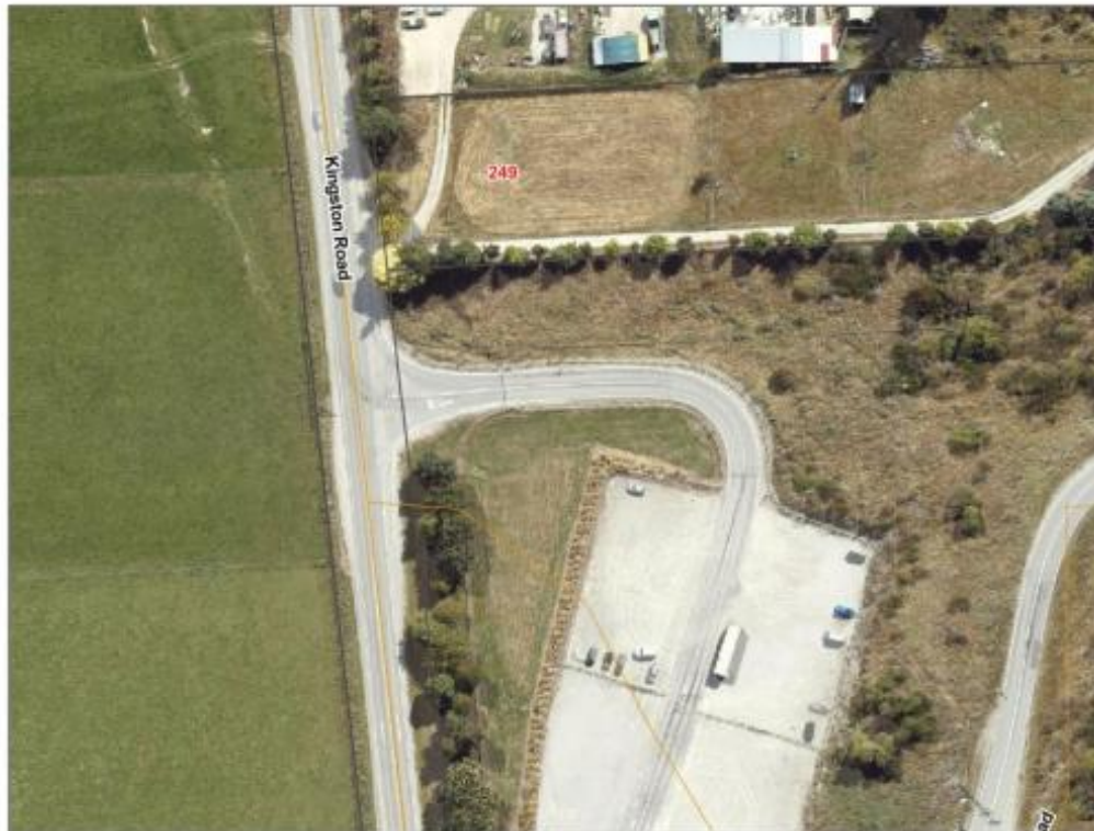
Figure 2-49: SH6 / Remarkables Ski Field Access Road.
