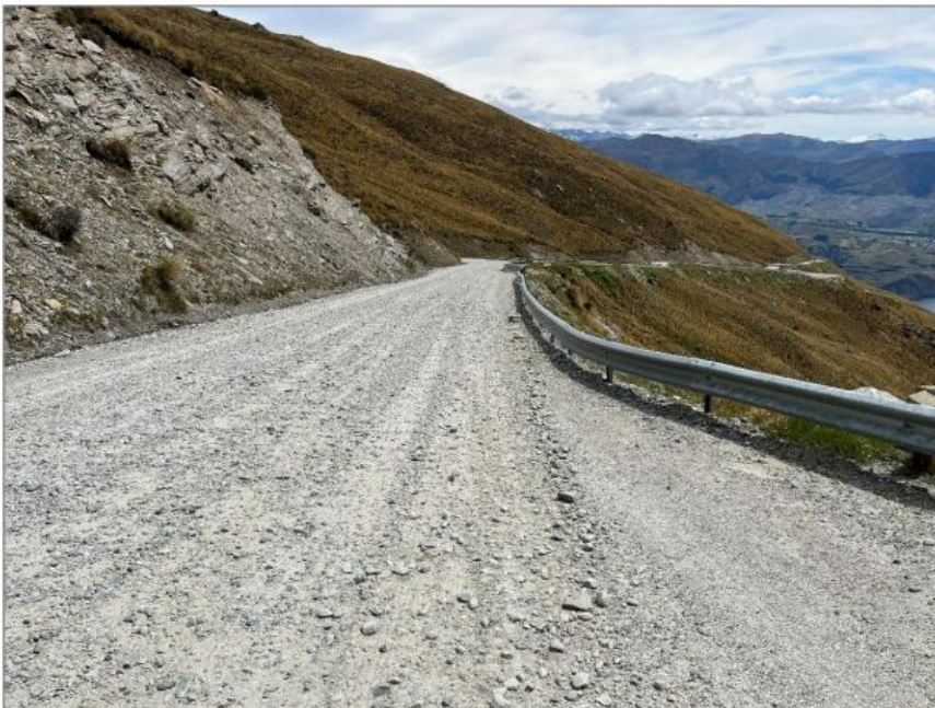
Figure 2-51: Typical view of Remarkables Ski Field gravelled section of the access road.
