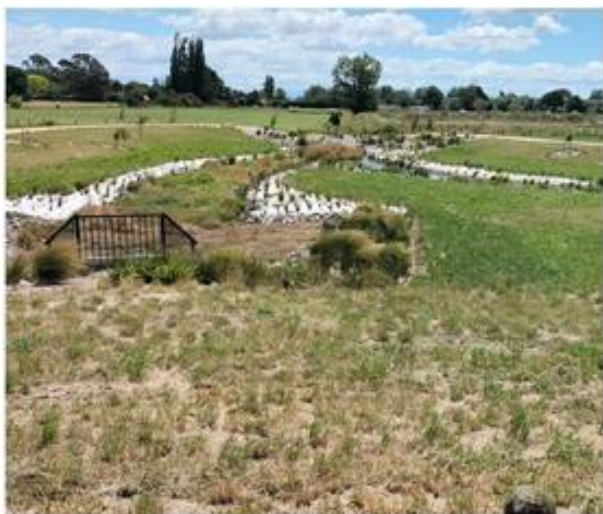
Figure 4: 148 Middle Road looking northwest, Iona stormwater pond in foreground
