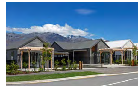
Image from JTB Architects, Tewa Banks
