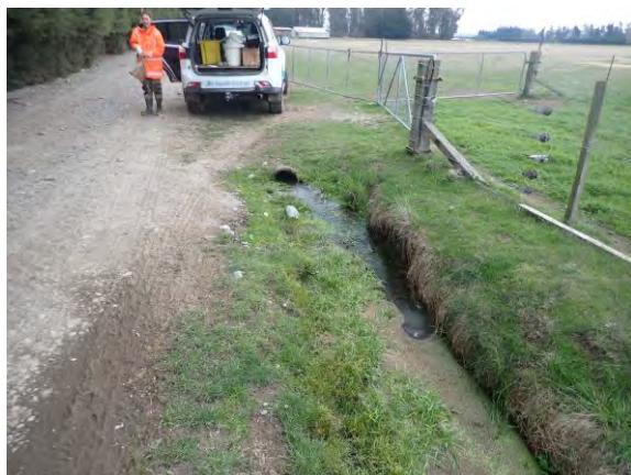
Figure 5a. Example of the small existing farm culverts, July 2024.
