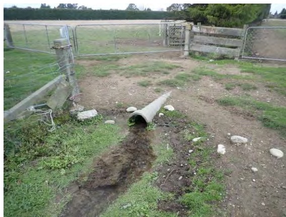
Figure 5b. Example of the small existing farm culverts, July 2024.
